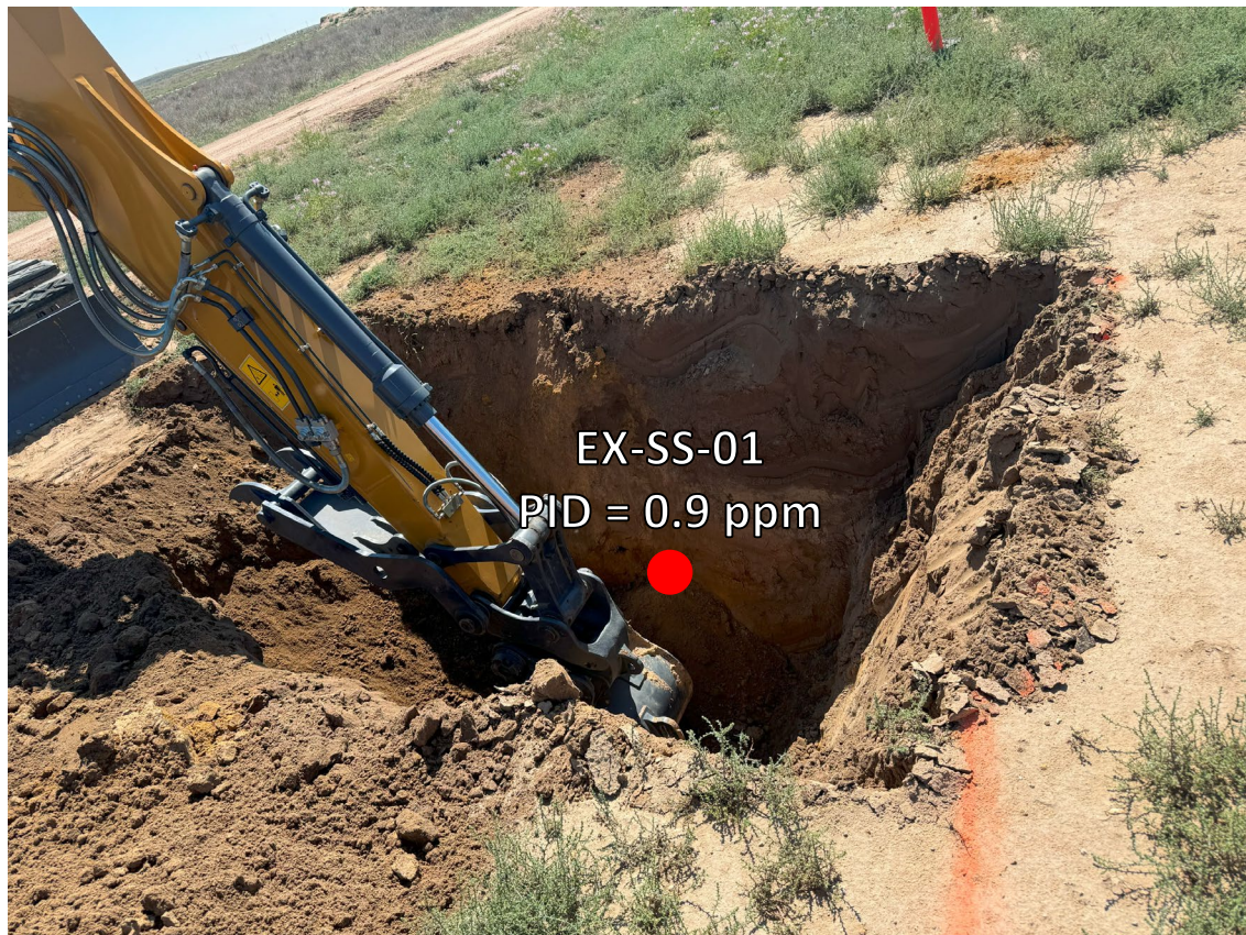
Looking southeast at former wellhead footprint
