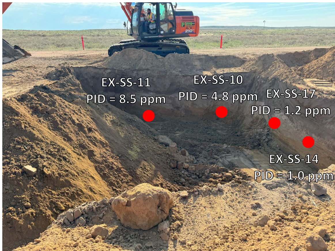
Looking east at former wellhead footprint
