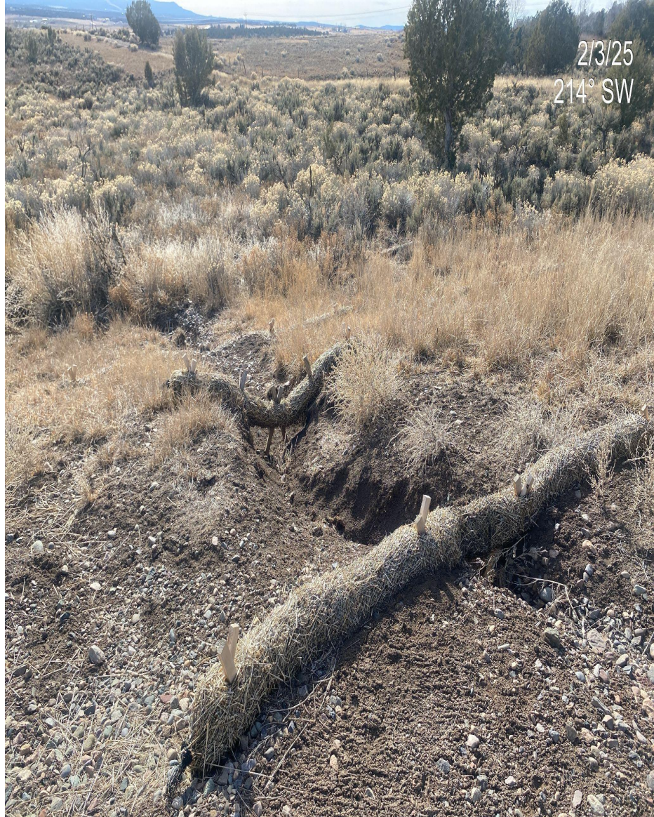
Photo 3. Stormwater issues persist in the southern interim reclamation area. BMPs have not been installed correctly.
