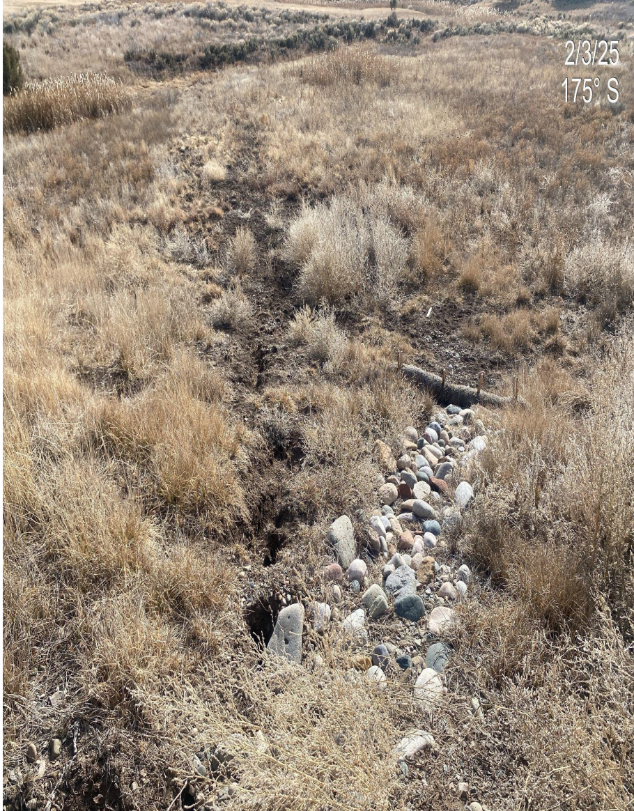
Photo 3. Stormwater issues persist in the southern interim reclamation area. BMPs have not been installed correctly.
