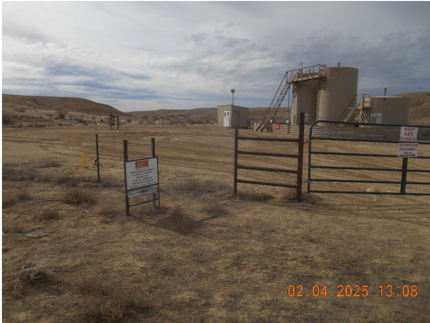
Location overview looking SW.
