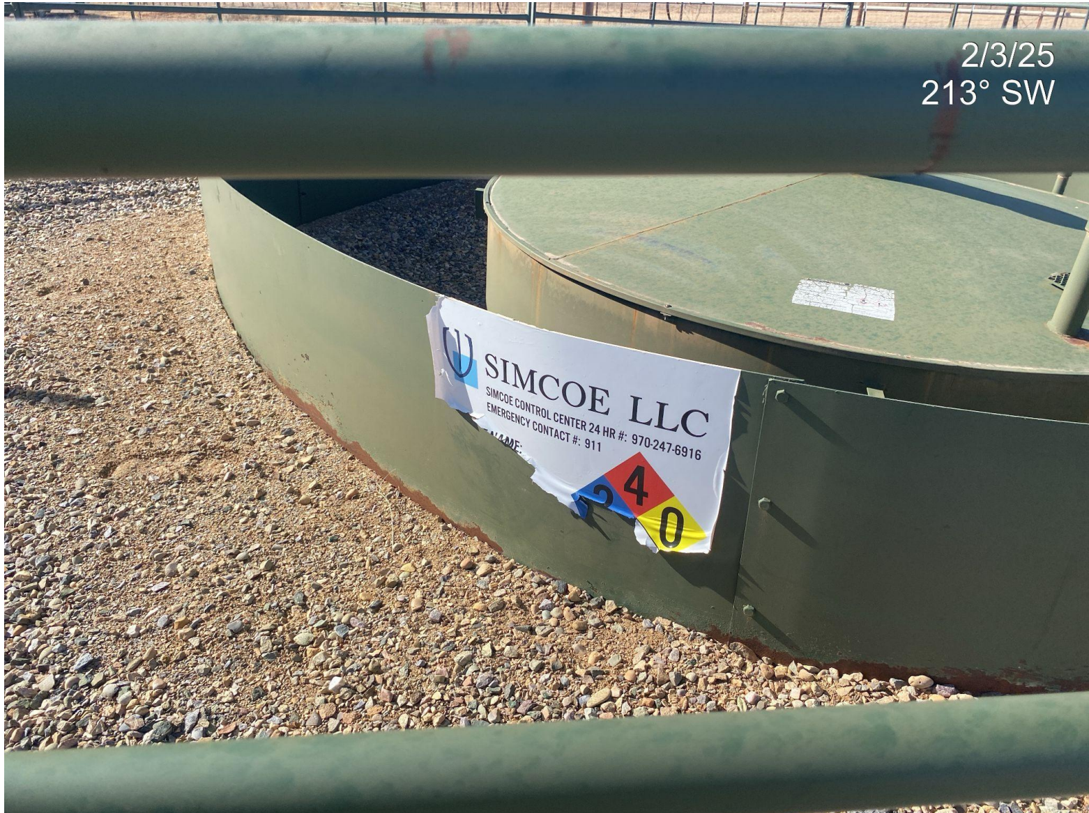
Photo 3. Produced water tank label has deteriorated and is no longer displaying tank capacity.
