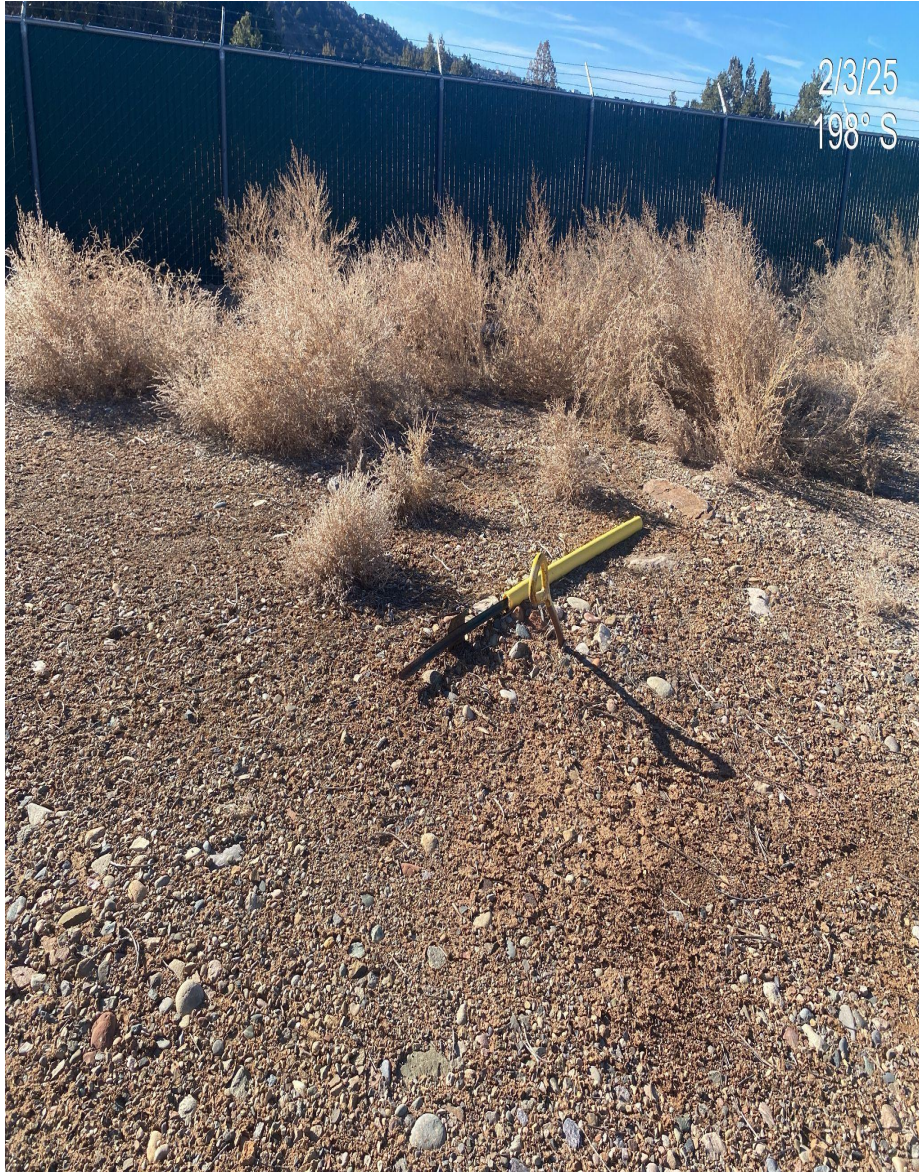
Photo 3. 2 unmarked guy line anchors on active pad.
