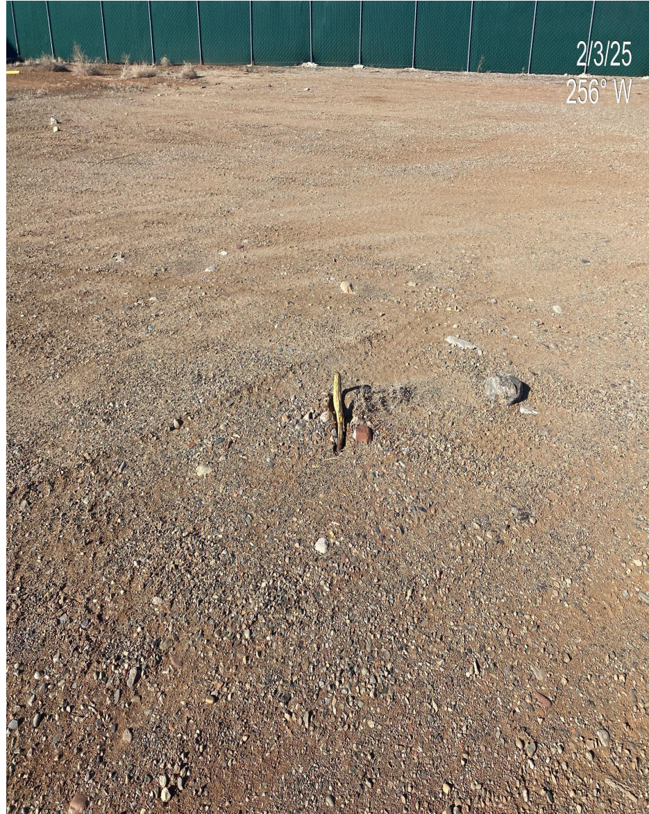
Photo 3. 2 unmarked guy line anchors on active pad.
