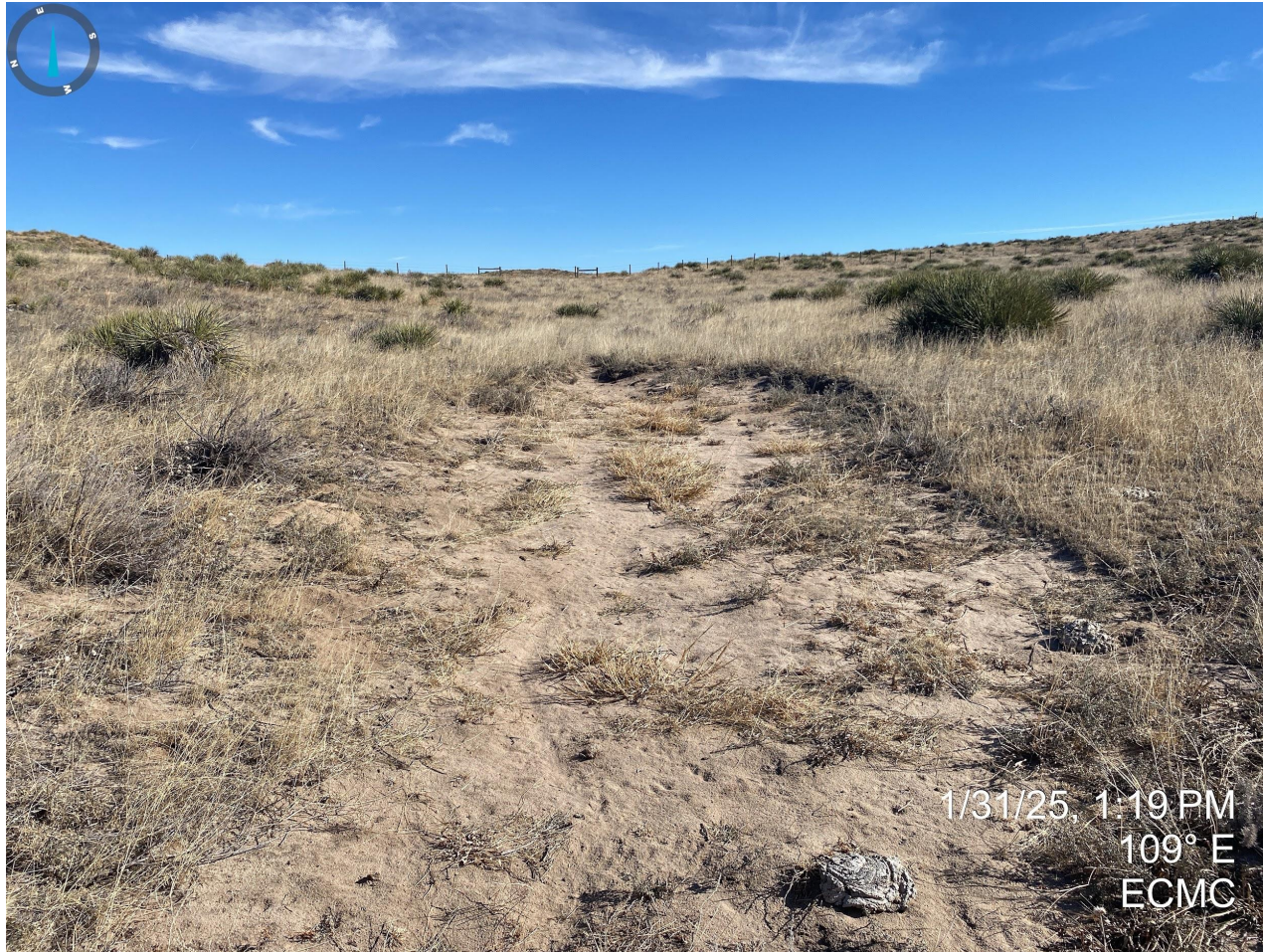
Photo 4. Taken along the access road. It does not appear that the access road has been reclaimed with evidence of non-uniform vegetation cover resulting in bare soil.
