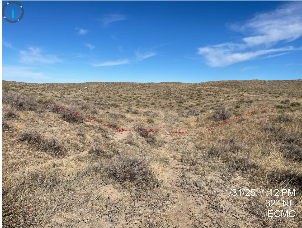
Photo 3. Taken along the access road. Red dotted line illustrates that a portion of the access road does not appear to have been recontoured to reflect adjacent topography.
