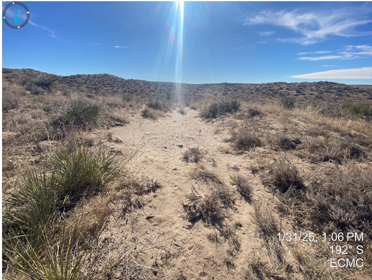
Photo 1. Taken near the start of the access road. It does not appear that the access road has been reclaimed with evidence of non-uniform vegetation cover resulting in bare soil.
