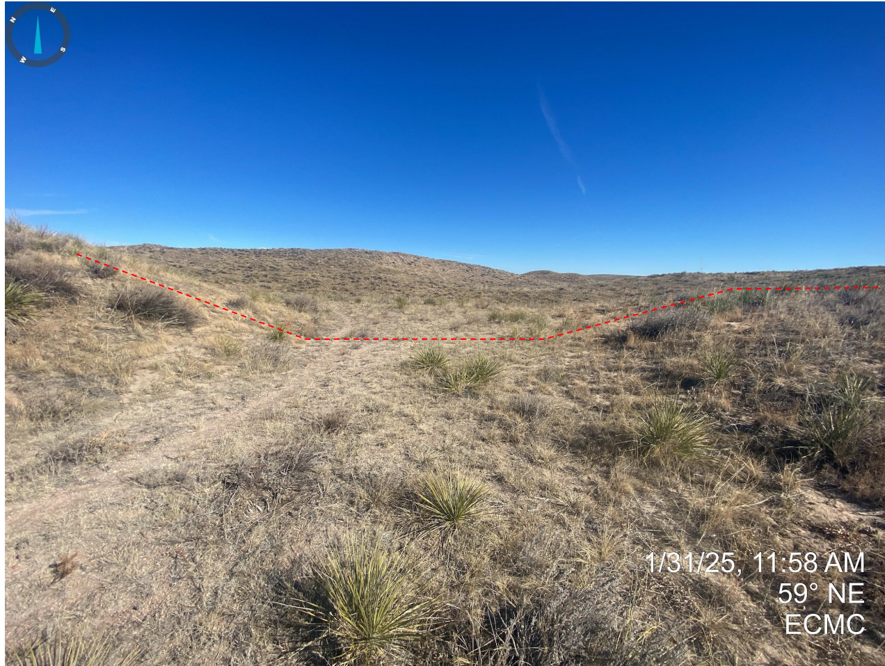
Photo 5. Taken along the access road. Red dotted line illustrates that the access road does not appear to have been recontoured to reflect adjacent topography.
