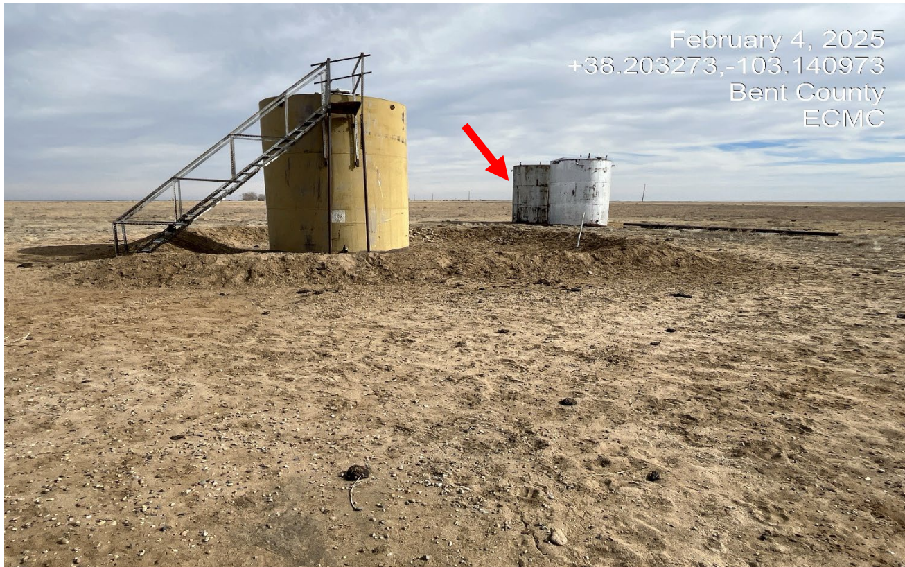
Photo 18. Facing southwest at the location. The old tank was removed and anew one has been installed. It is unknown if impacts around the tank were cleaned up. There are two unused tanks stored on location at red arrow.
