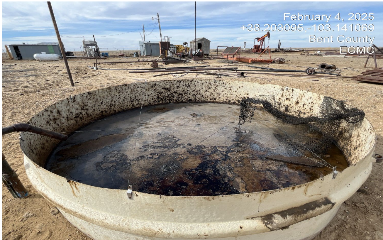
Photo 20. Facing toward the open top tank which has oil condensate inside the tank with no wildlife or livestock protection.
