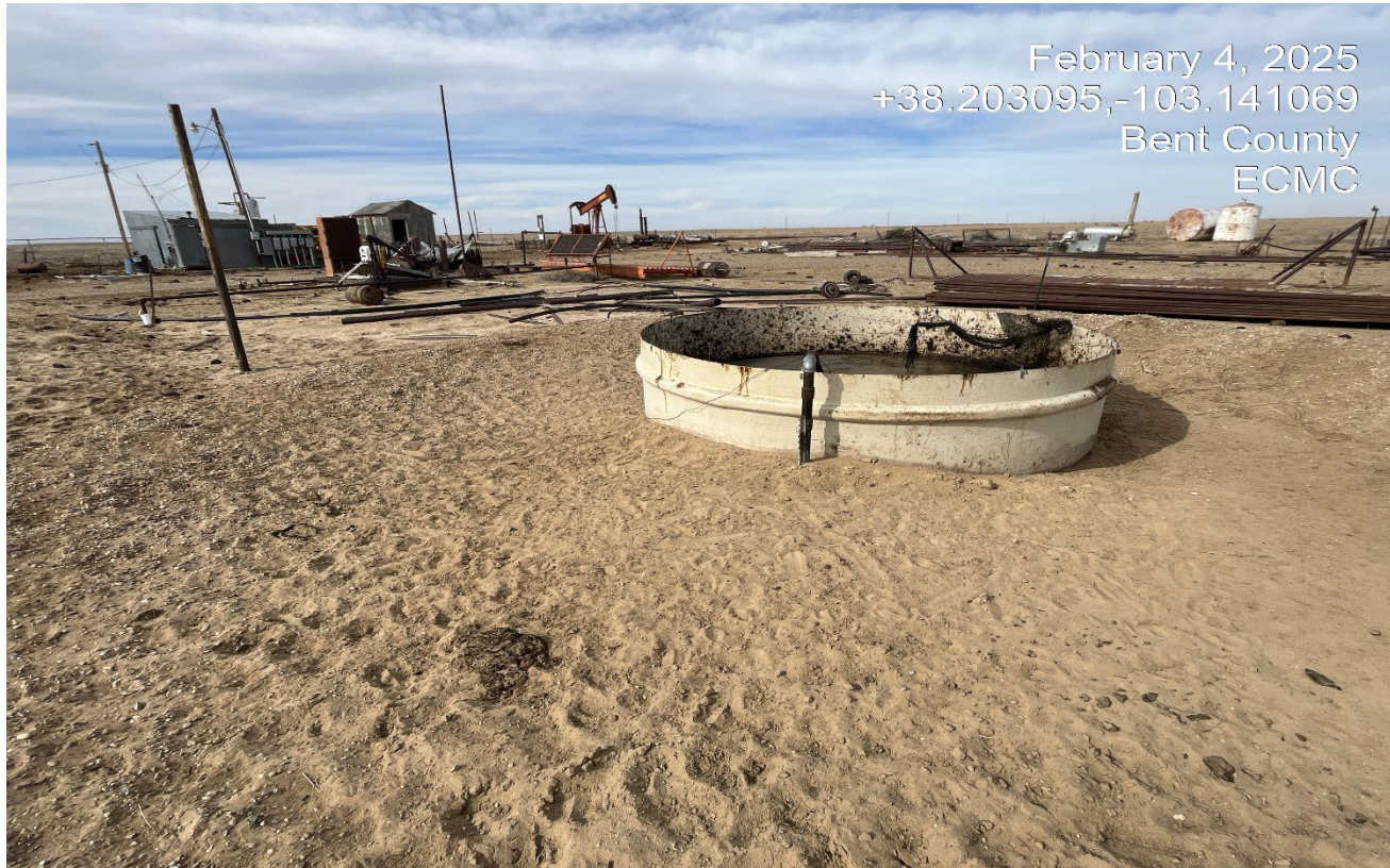
Photo 19. Facing northwest at the south side of the location. There is an open top fiberglass condensate tank with no wildlife or livestock protections. There are cattle tracks all around the tank indicating that cattle could be drinking out of this tank.
