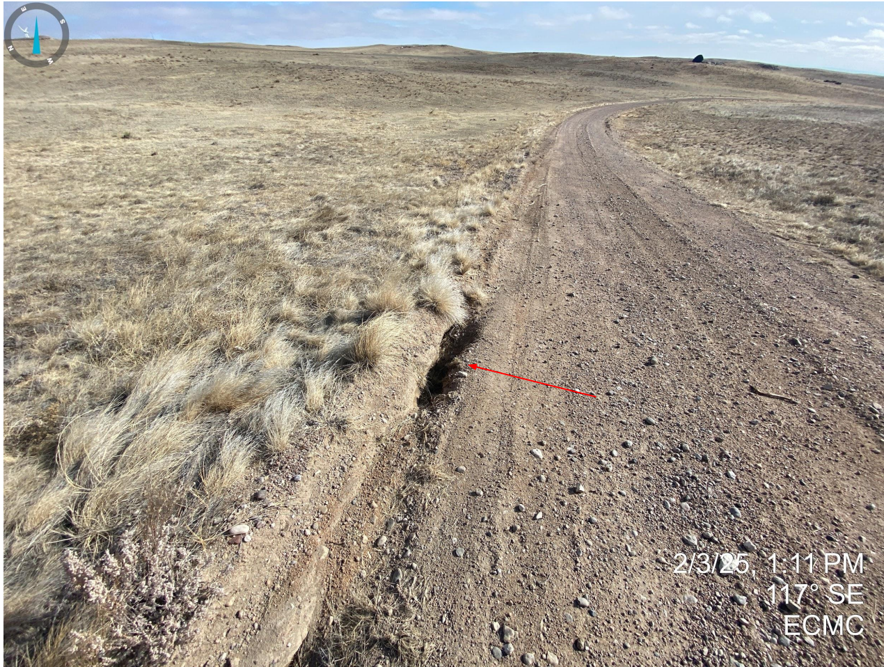
Photo 20. Continued from Photo 19. While some work appears to have been completed to repair erosion degradation along the northern portion of the access road, there is still evidence of erosion degradation that requires maintenance.
