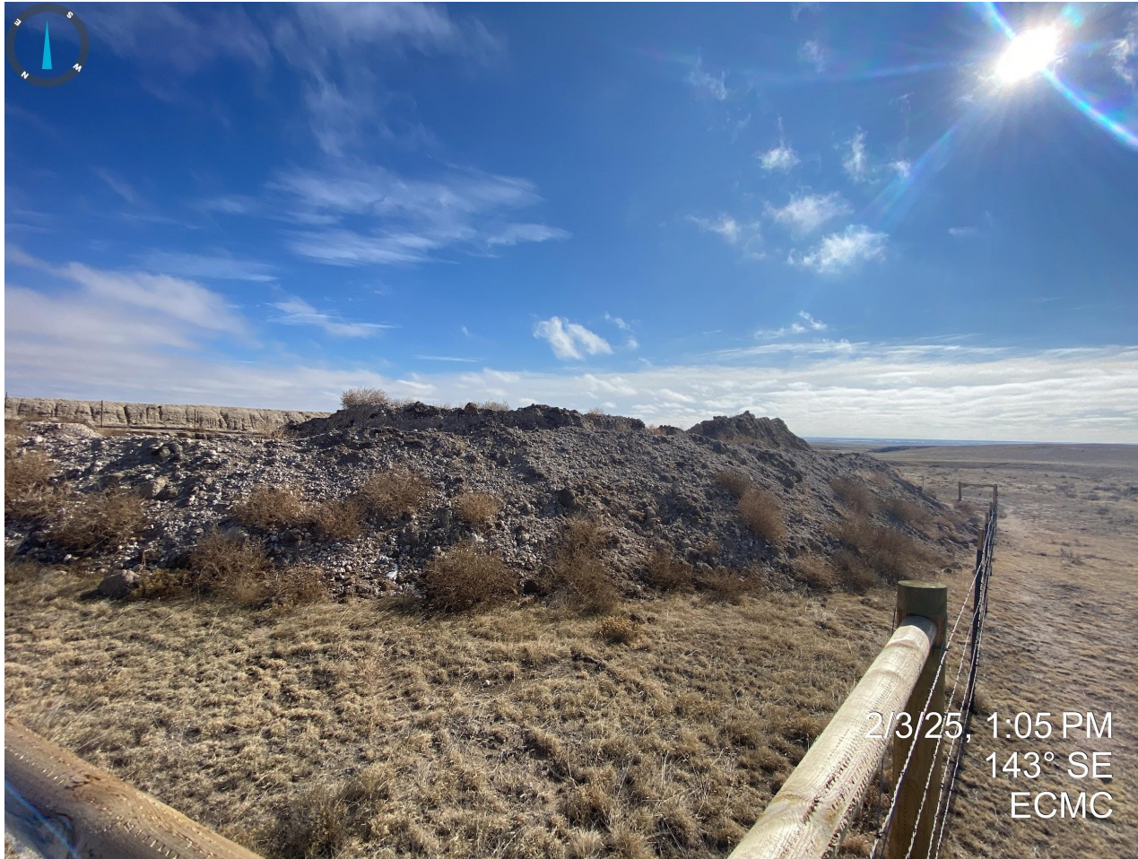
Photo 1. Taken from the north side of the stockpiled soils. No perimeter stormwater control measures/BMPs, or impermeable liners underneath the stockpile were observed. Impacted soils appear to have been placed directly on top of undisturbed lands. Additionally, it does not appear that topsoil has been salvaged Per Rule 1002.b prior to stockpiling the soil on undisturbed portions of land. Undesirable vegetation observed throughout stockpiled areas.
