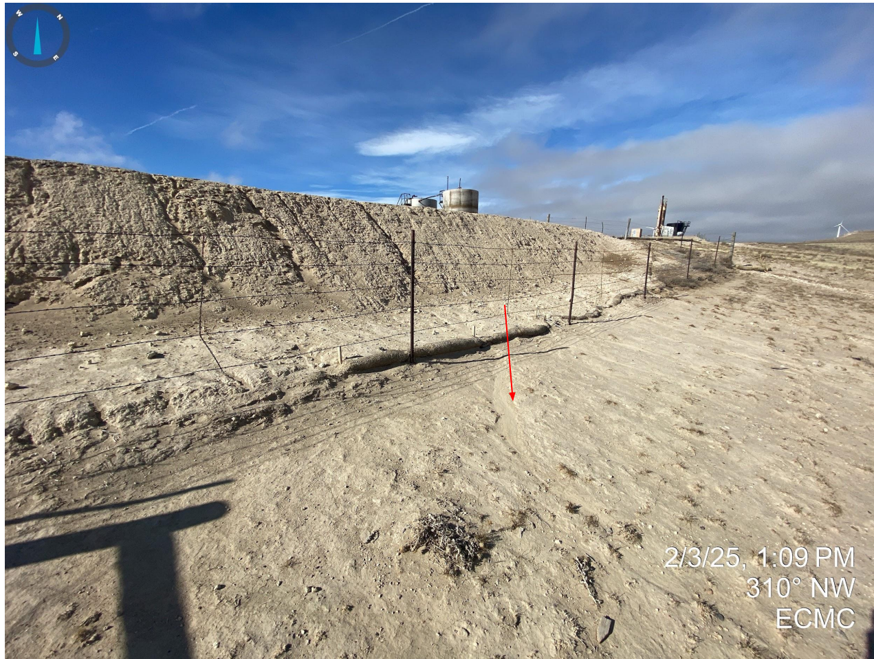
Photo 11. Continued from Photo 10. New stormwater erosion degradation observed east of the pit. Stormwater control measures remain inadequate.
