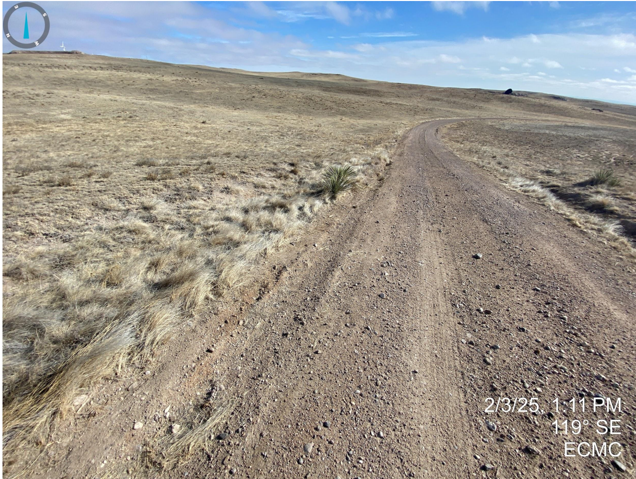
Photo 19. It appears that erosion degradation along the north side of the access road has been repaired. See proceeding photo for additional information.
