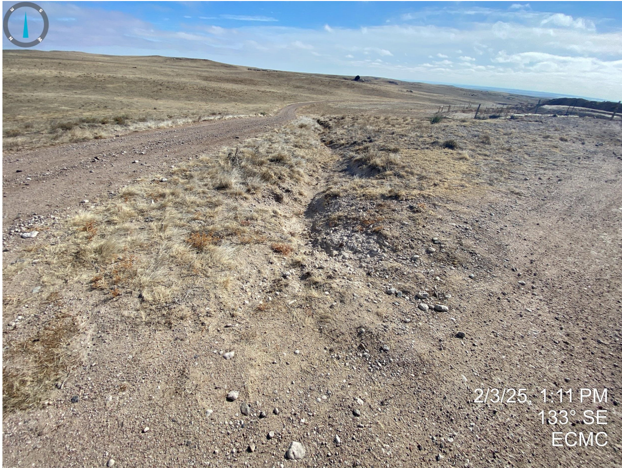
Photo 17. Taken north of pit. Evidence of erosion degradation, previously documented, does not appear to have been repaired/stabilized with no evidence of control measures/BMPs observed that would prevent further erosion of the production areas and access roads.
