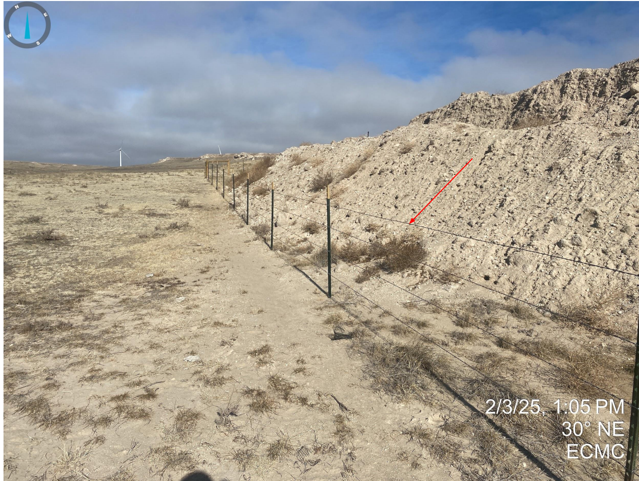
Photo 3. Continued from Photo 2; facing northeast. Evidence of unstabilized soils (rill erosion) and sediment migration outside of the fenced portions. Undesirable vegetation (russian thistle) also observed.
