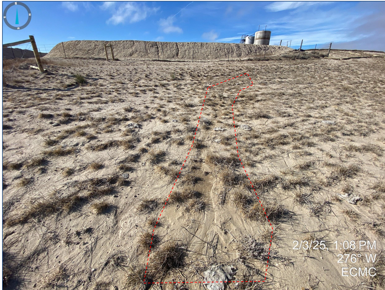
Photo 10. New stormwater erosion degradation observed east of the pit. Stormwater control measures remain inadequate.
