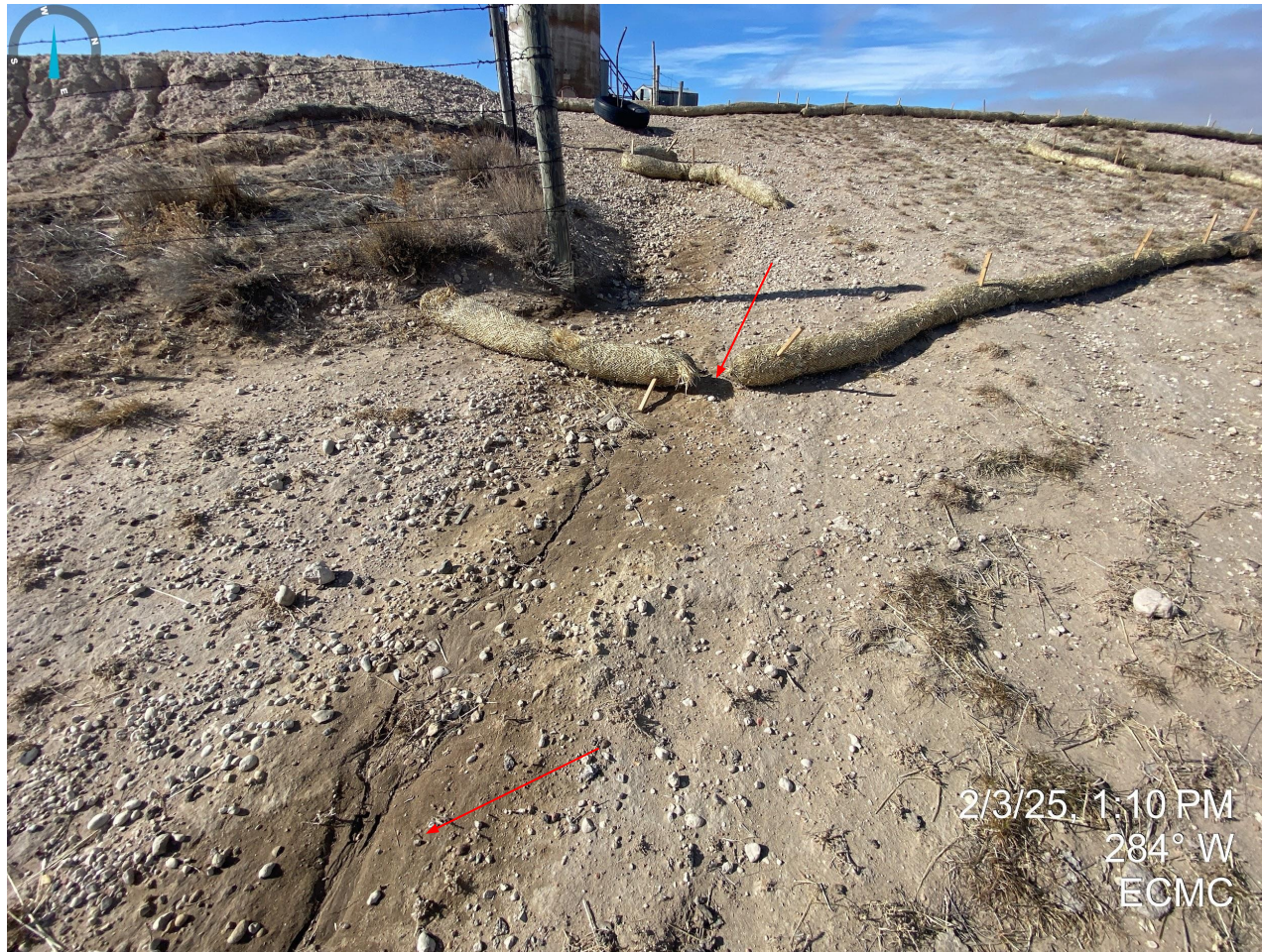
Photo 14. Erosion degradation occurring on the northern/eastern portion of the production areas, near the pit. Stormwater control measures appear to be degraded/damaged and not properly functioning with erosion degradation evidence.
