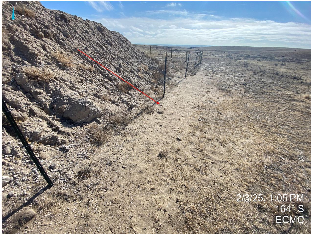
Photo 2. Continued from Photo 1; evidence of unstabilized soils (rill erosion) and sediment migration outside of the fenced portions. Undesirable vegetation (russian thistle) also observed.
