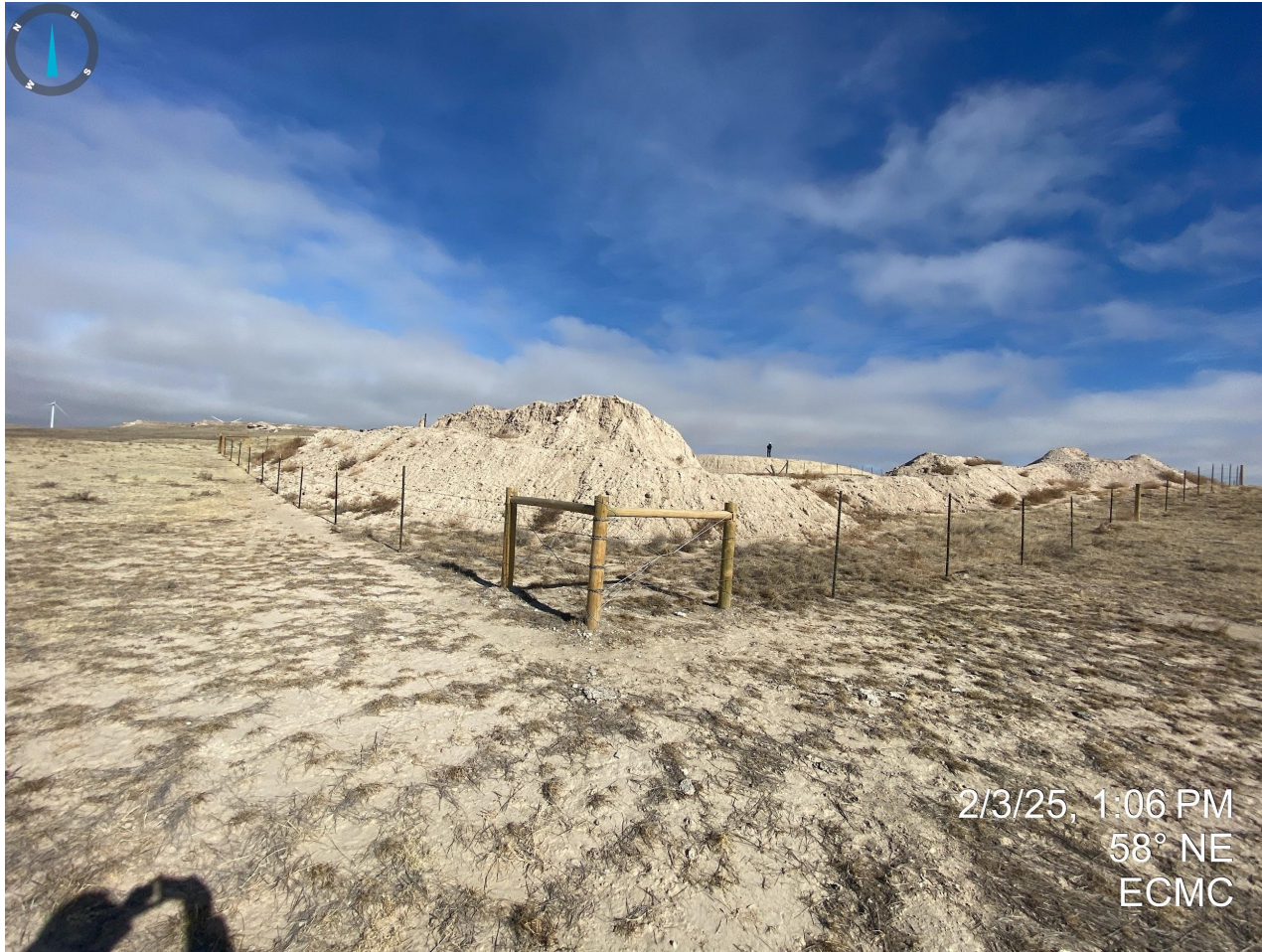
Photo 4. Sediment deposition resulting from unstabilized stockpiles, southwest corner of the pit.
