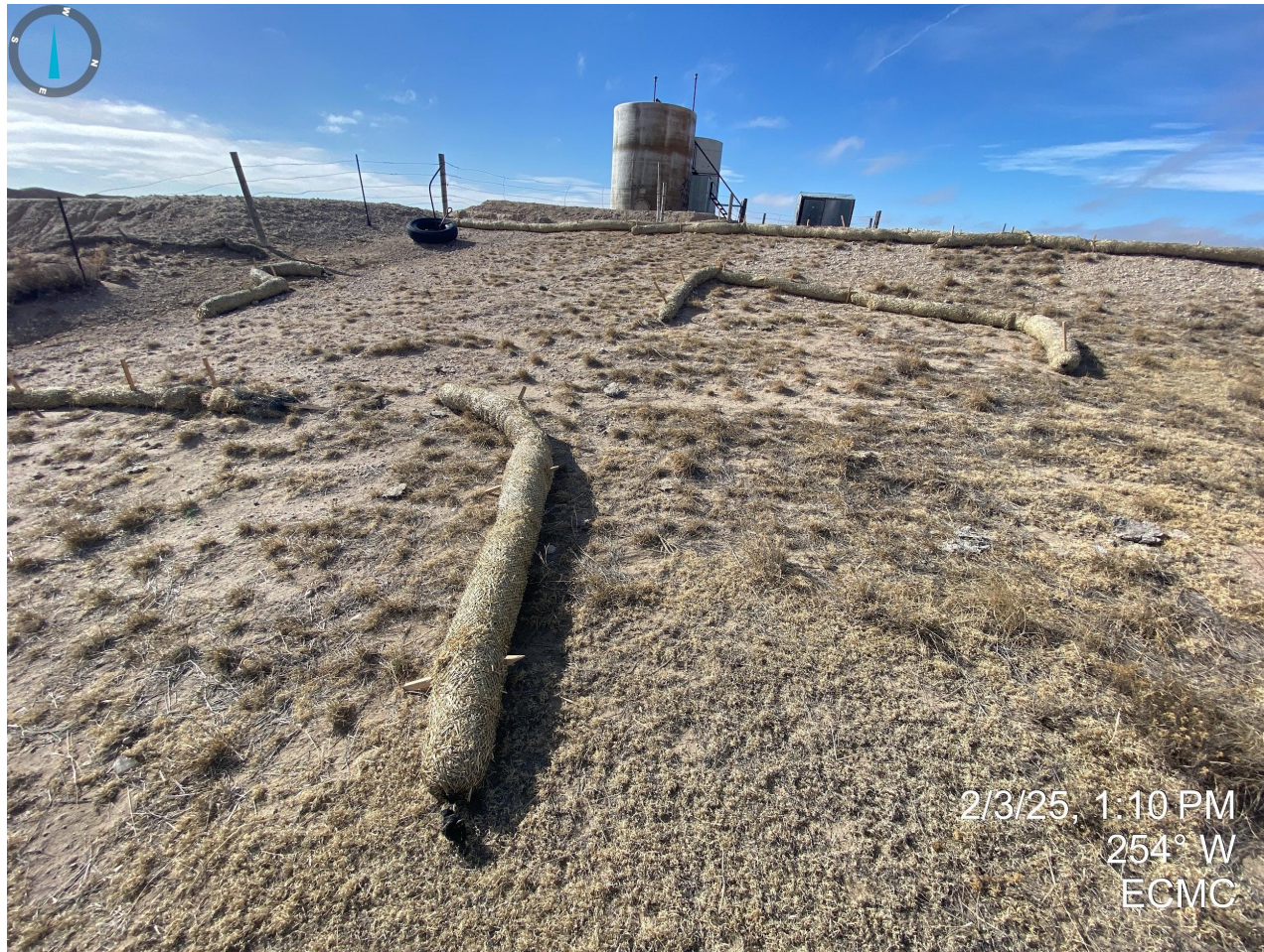
Photo 16. Northern/eastern portion of the production areas, near the pit. Stormwater control measures do not appear to be installed per good engineering practices.
