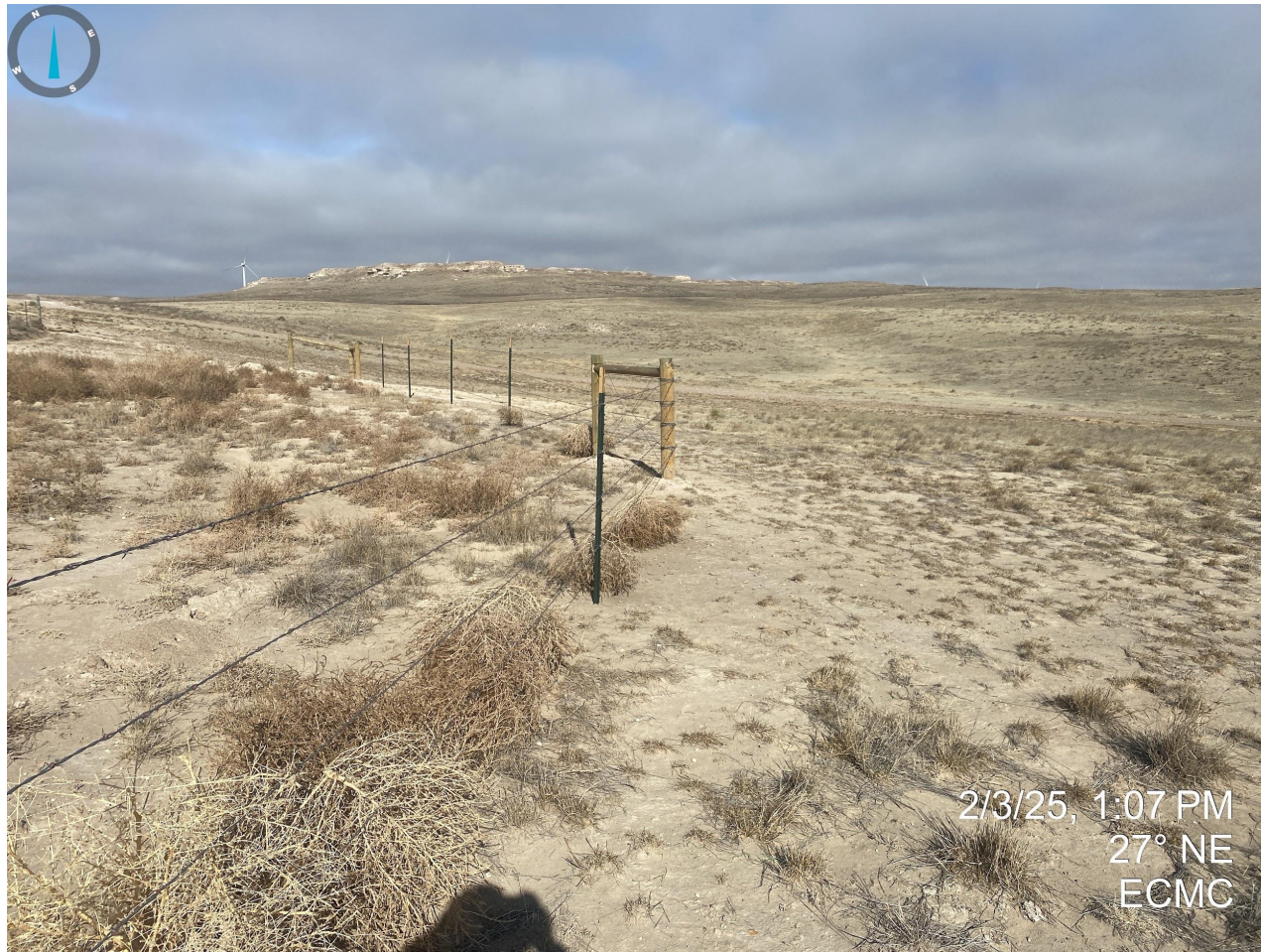
Photo 7. Taken southeast of the excavated area and stockpiled material; no apparent perimeter stormwater control measures and sediment deposition observed. Tumbleweed debris also pictured.
