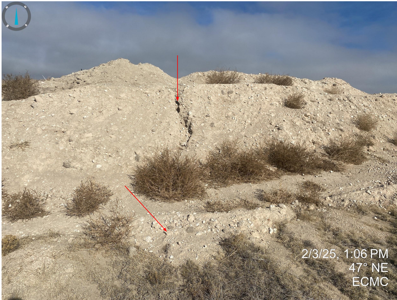
Photo 5. Evidence of erosion degradation and sediment migration from the unstabilized stockpiles. Also pictured, russian thistle/tumbleweed debris. South side of stockpiles.
