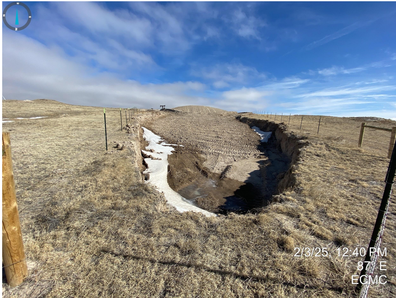
Photo 6. Western extent of excavation. It appears that stockpile (background) has been equipment tracked for short term stabilization and the excavation has been roughened. Undesirable vegetation previously documented appears to have been removed.
