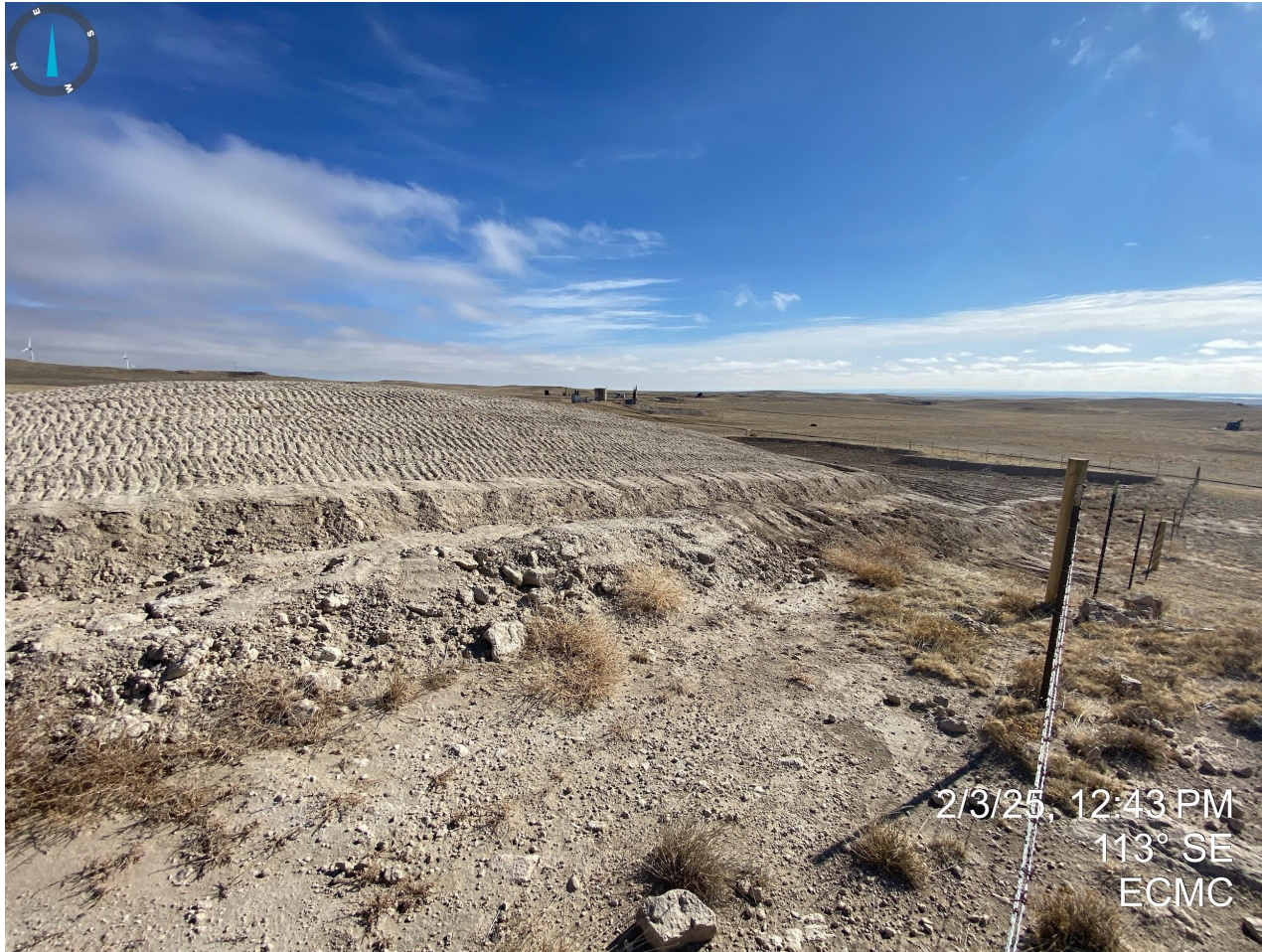
Photo 10. Southern/eastern salt kill excavation. It appears that a berm has been constructed around the stockpile, which has been equipment tracked for short term stabilization.
