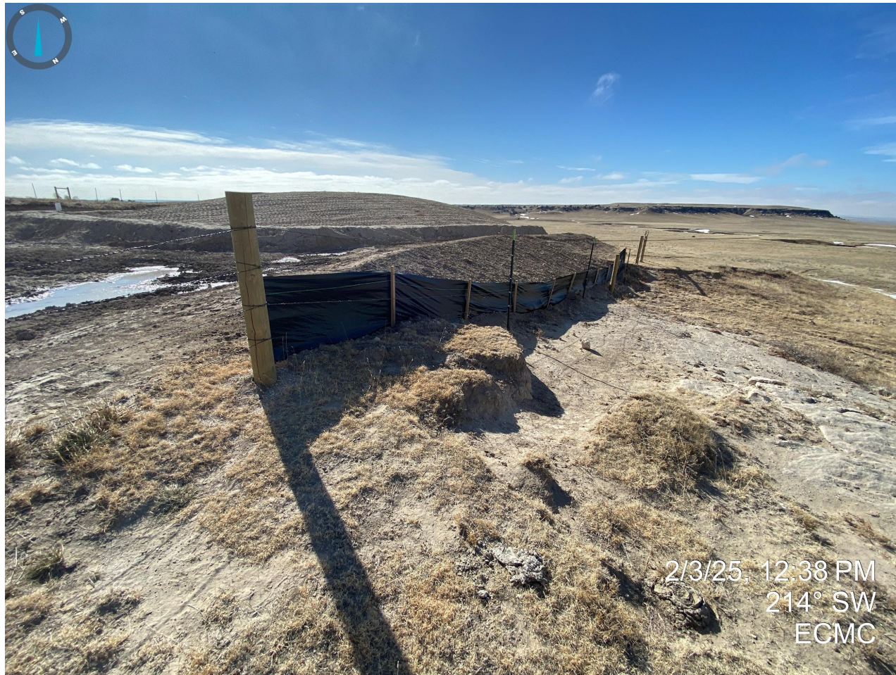
Photo 3. Additional stormwater and erosion control BMPs (silt fence) appear to have been implemented on the north/west side of the pit near the adjacent drainage.
