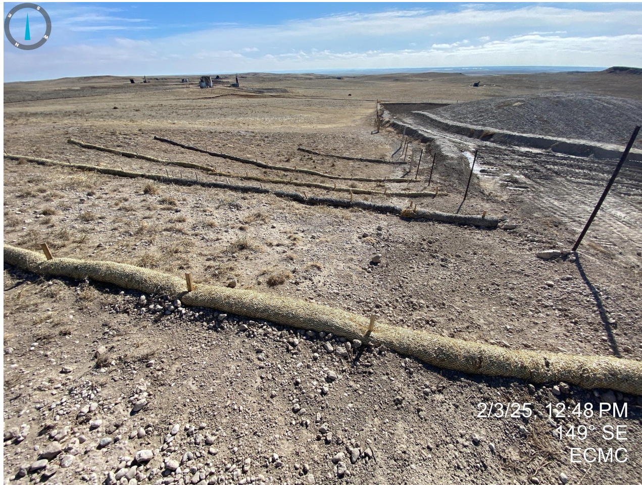
Photo 15. Eastern side of pit. It appears that erosion degradation has been repaired and stormwater control measures installed per good engineering practices. Additional reclamation activities are required to stabilize areas experiencing bare soil and/or non-uniform vegetation cover.
