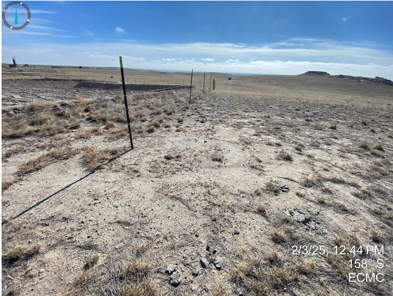
Photo 11. Southern/eastern salt kill excavation. Additional reclamation activities are required to stabilize areas experiencing bare soil and/or non-uniform vegetation cover.
