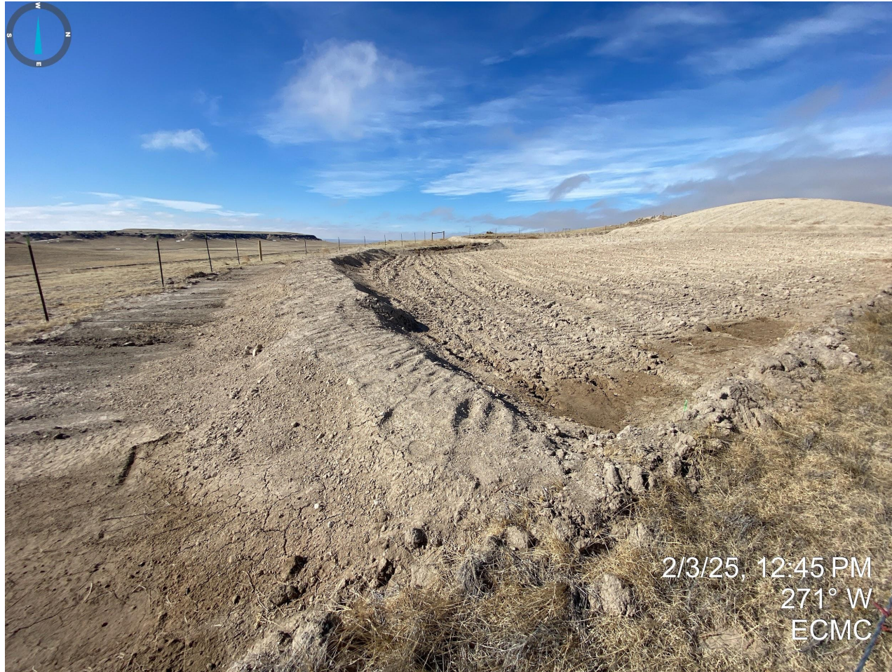
Photo 12. Southern/eastern salt kill excavation. A berm has been constructed at the southern portion of the excavation. Undesirable vegetation previously documented also appears to have been removed.
