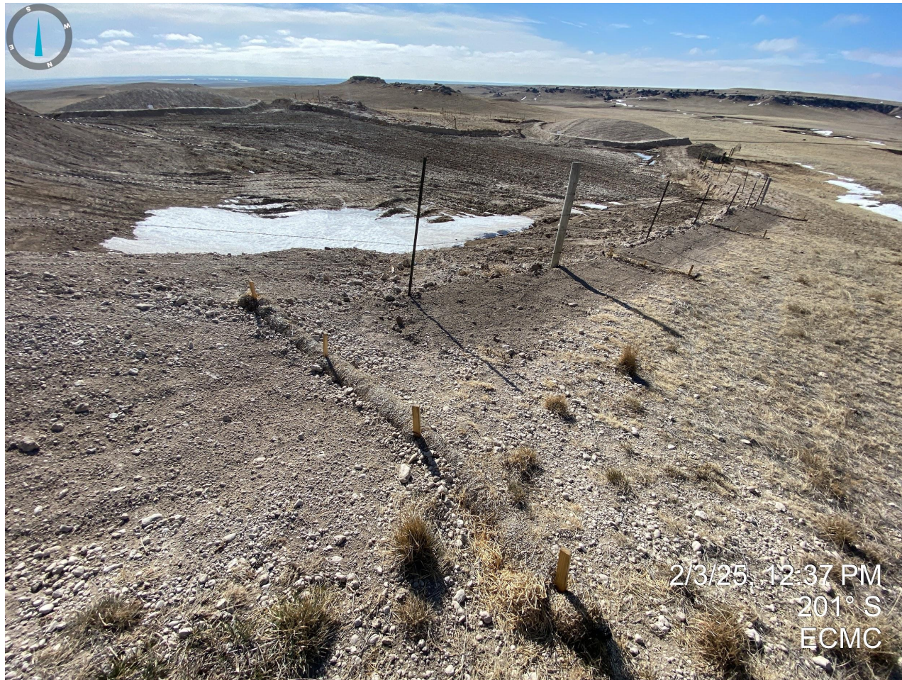
Photo 2. North side of pit. Straw wattles appear to have been installed per good engineering practices (trenched and backfilled). Additional reclamation activities are required to stabilize the bare/exposed soils.
