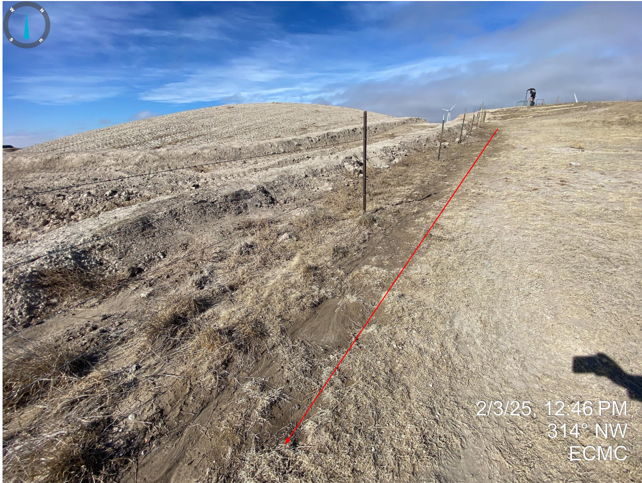
Photo 13. Southern/eastern salt kill excavation, east side. Erosion degradation from lack of proper stormwater control measures.
