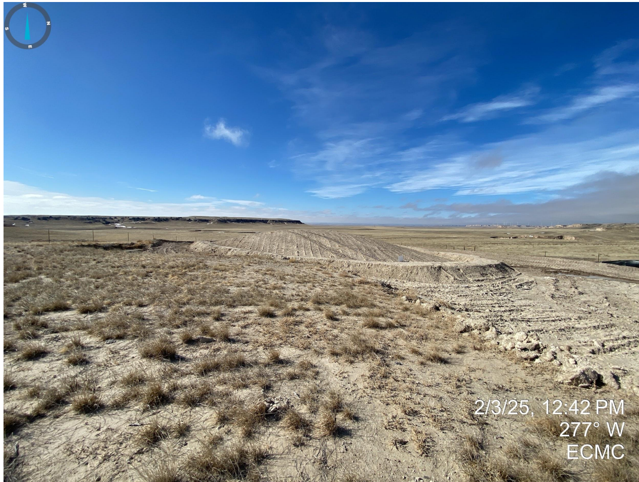
Photo 8. Photo taken between the two stockpiles, south side of pit excavation. Additional reclamation activities are required to stabilize areas experiencing bare soil and/or non-uniform vegetation cover.
