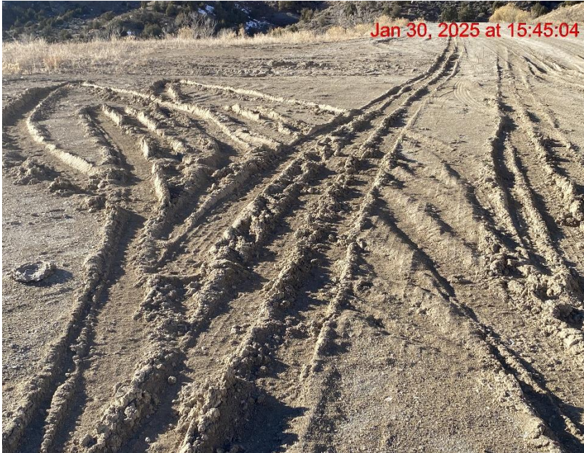
Lack of Stabilization – Photo #06392
