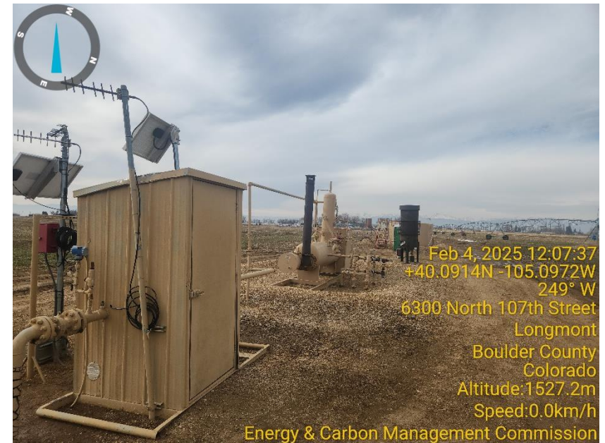
Photo 8 ECD, horizontal heated separator & gas meter run.
