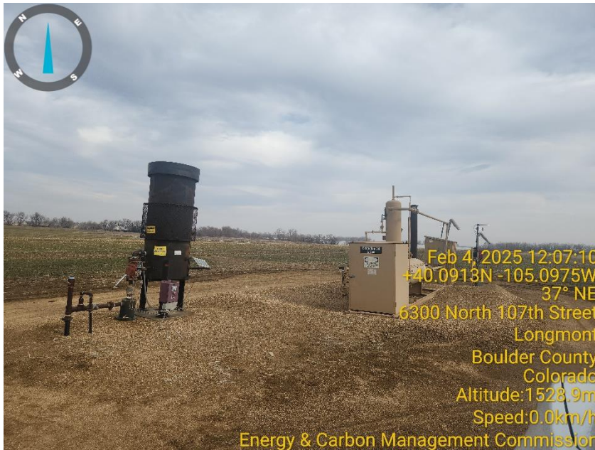
Photo 7 ECD, horizontal heated separator & gas meter run.
