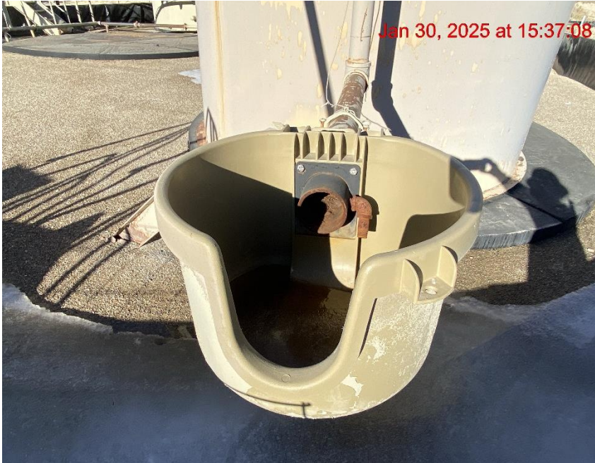
Open-Ended Load Line – Photo #06378
