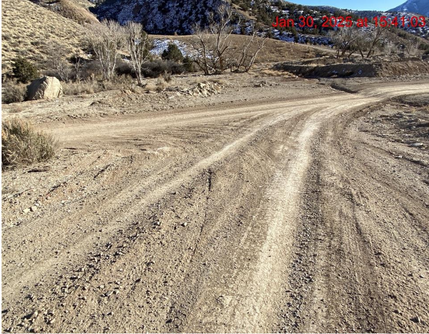
Insufficient Tracking BMPs – Photo #06384
