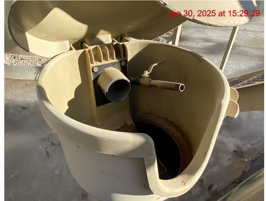
Open-Ended Load Line – Photo #06371
