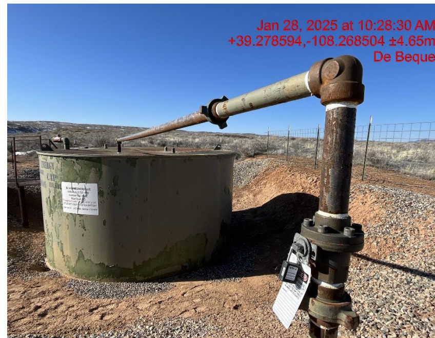
Photo # 3610 Tank is empty and locked/tagged out, hole is still in tank and lacks integrity
