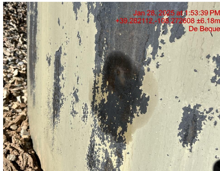
Photo # 3707 Suspected leaks on production tank/tank appears to lack integrity
