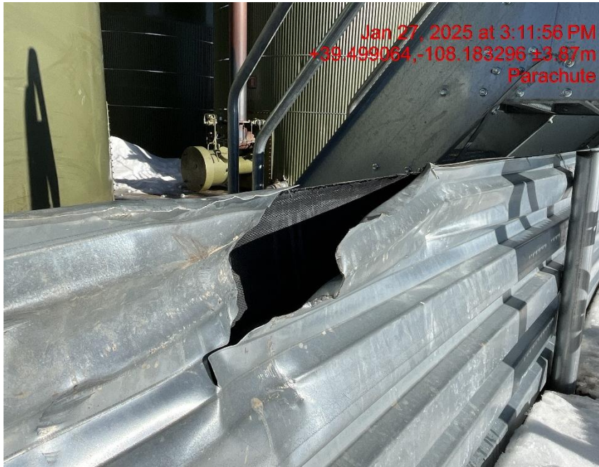
Photo # 3591 Containment showing signs of disrepair
