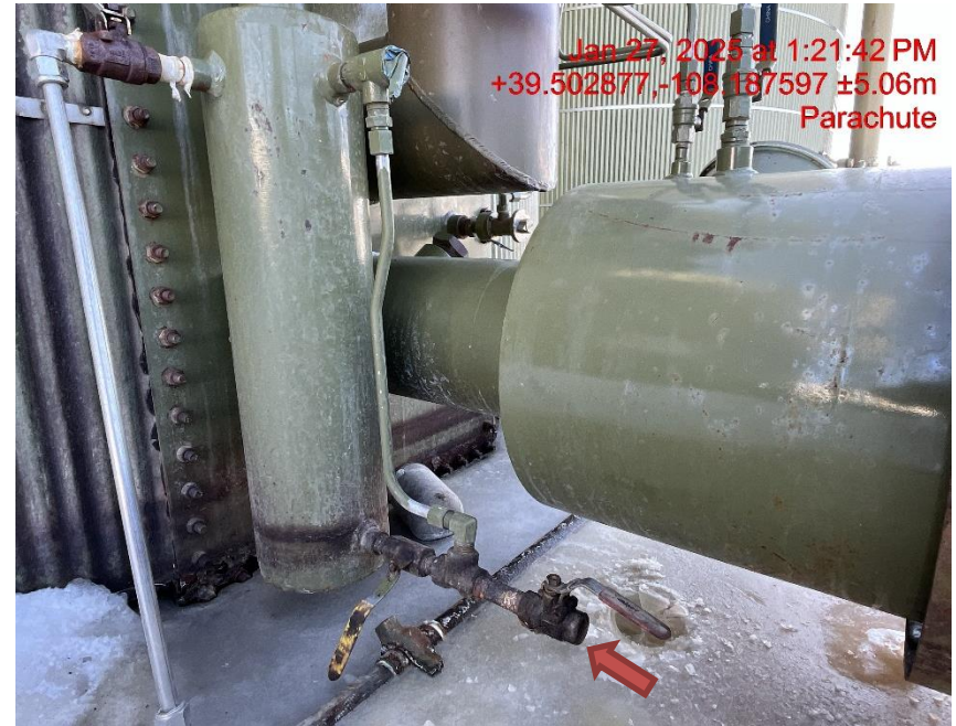
Photo # 3497 PRV vent line does not comply with CECMC pressure safety device rules
