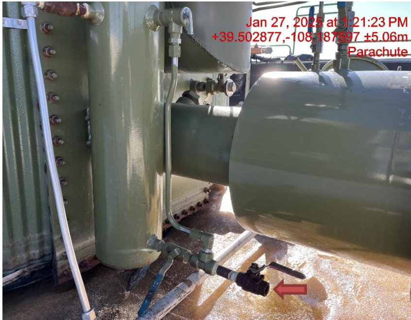
Photo # 3496 PRV vent line does not comply with CECMC pressure safety device rules
