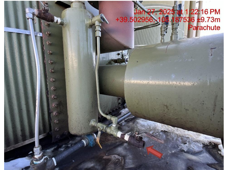
Photo # 3499 PRV vent line does not comply with CECMC pressure safety device rules
