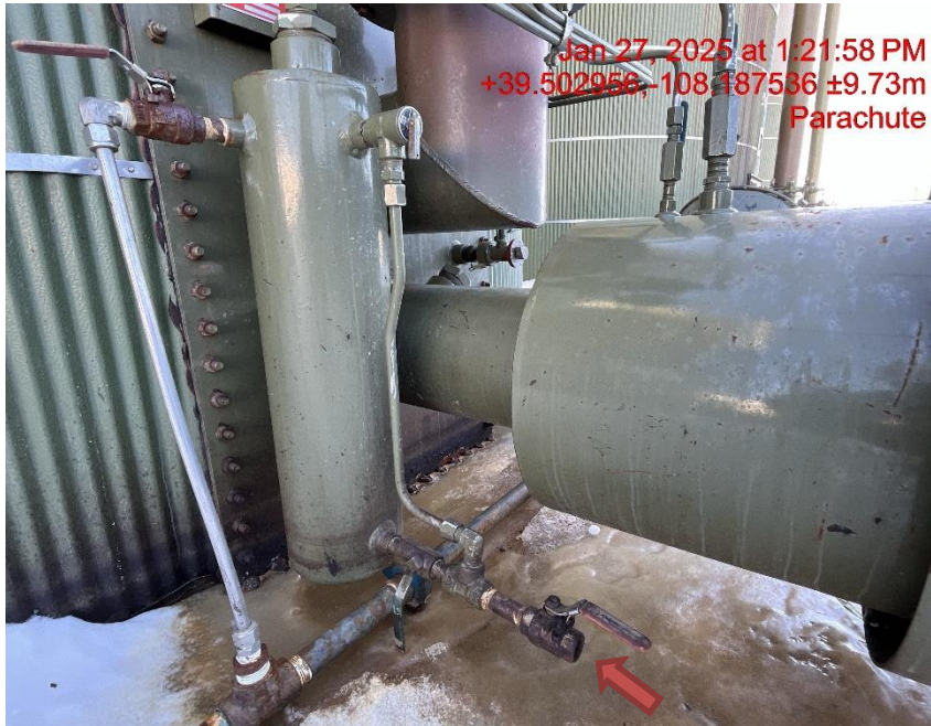
Photo # 3498 PRV vent line does not comply with CECMC pressure safety device rules
