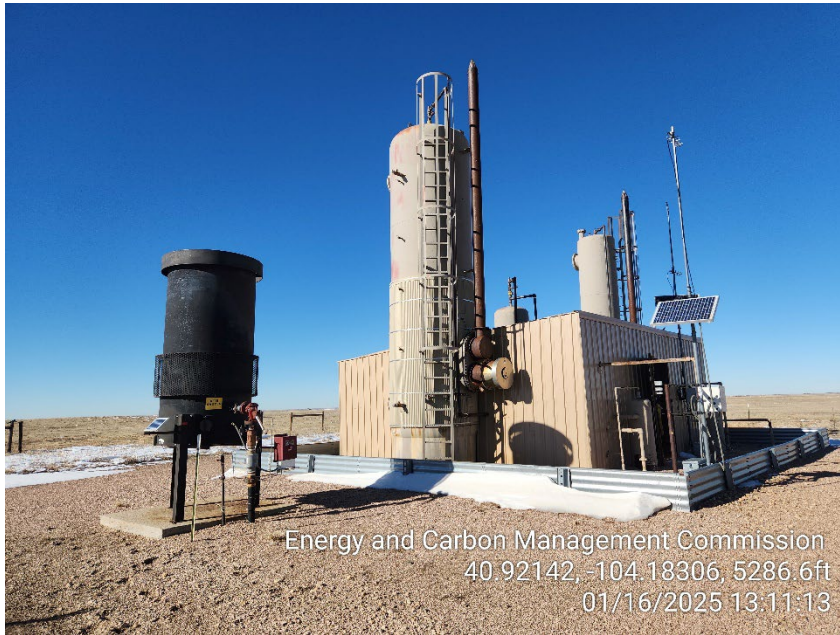
Photo 3 – Heater Treaters and ECDs
