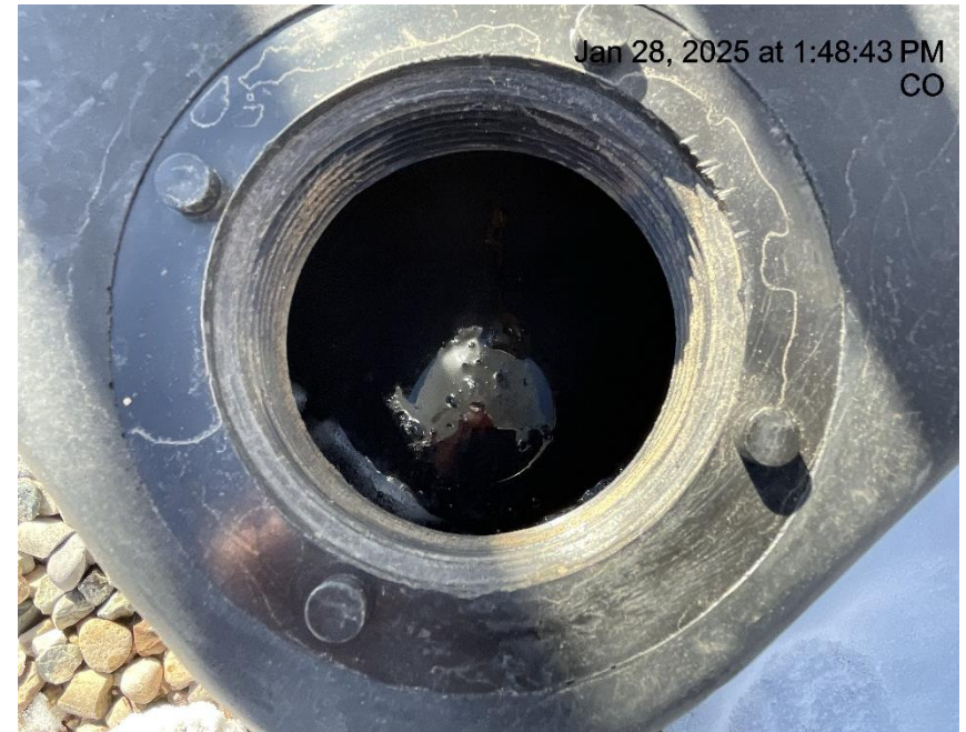
Photo # 1885 Failure to maintain chemical BMP – Chemical tank containment approximately 2/3 full of fluid/BMP insufficient to contain possible spill
