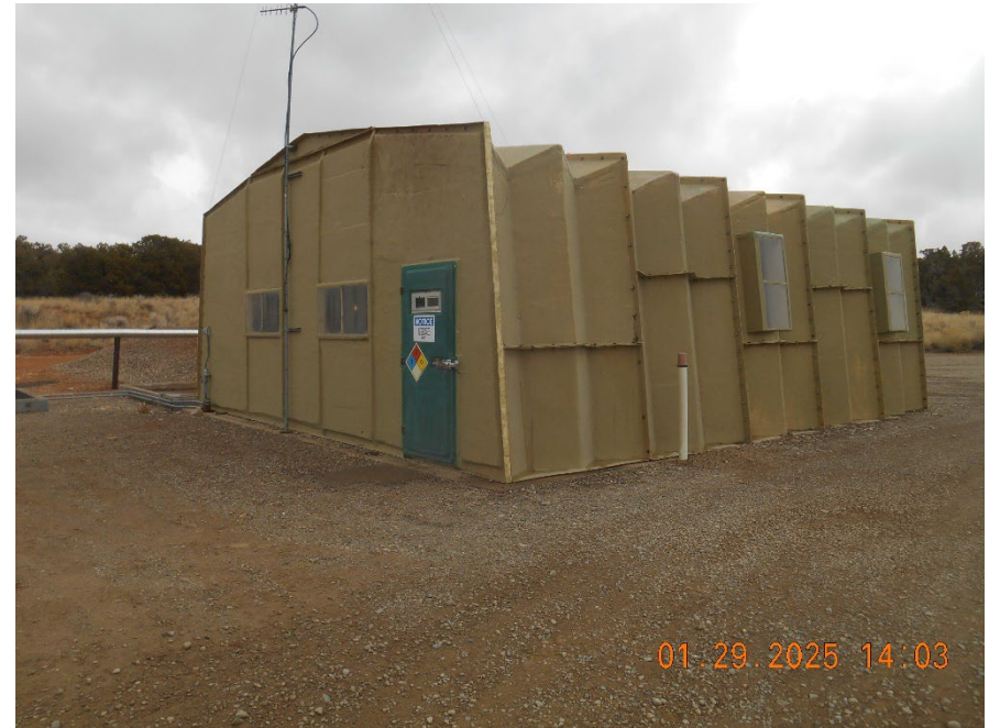
Manifold Housing and control station
