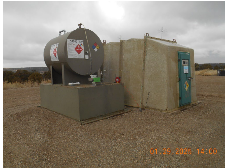
Injection wellhead housing Secondary containment of chemicals
