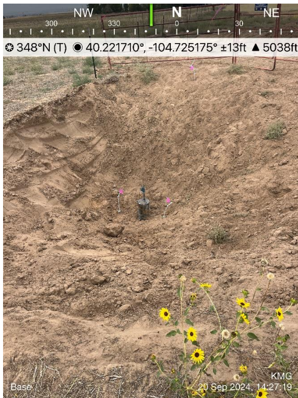
Wellhead Excavation
