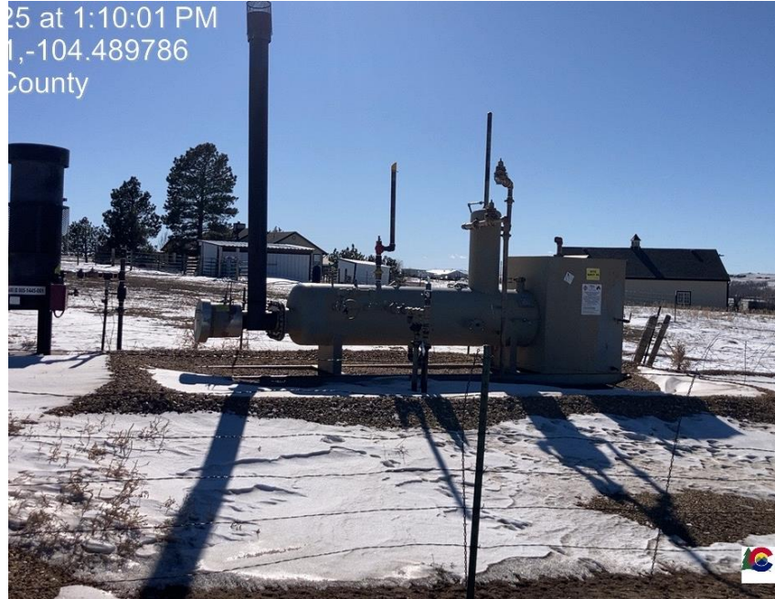
Pic 1 ECD, Separator
