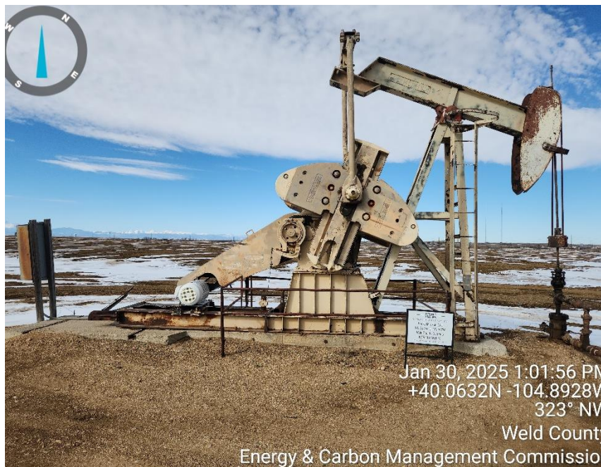
Photo 1 well head and equipment
