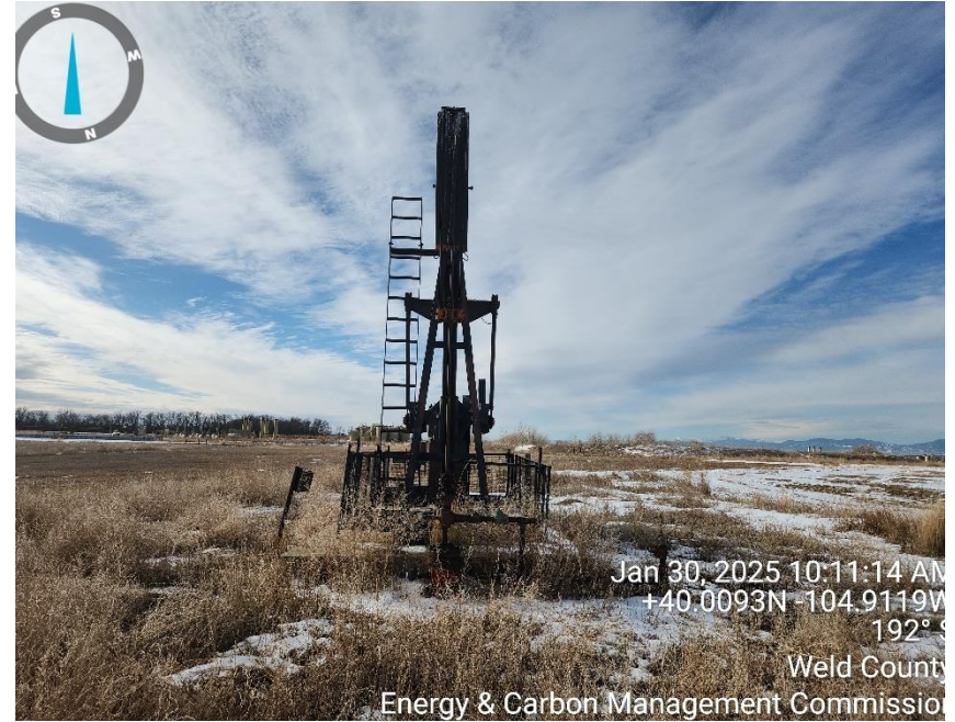
Photo 2 well head and equipment
