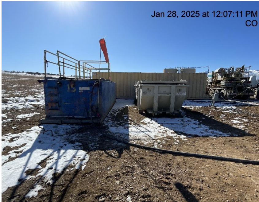
Photo # 1723 Tanks lack secondary containment/failure to comply with COA
