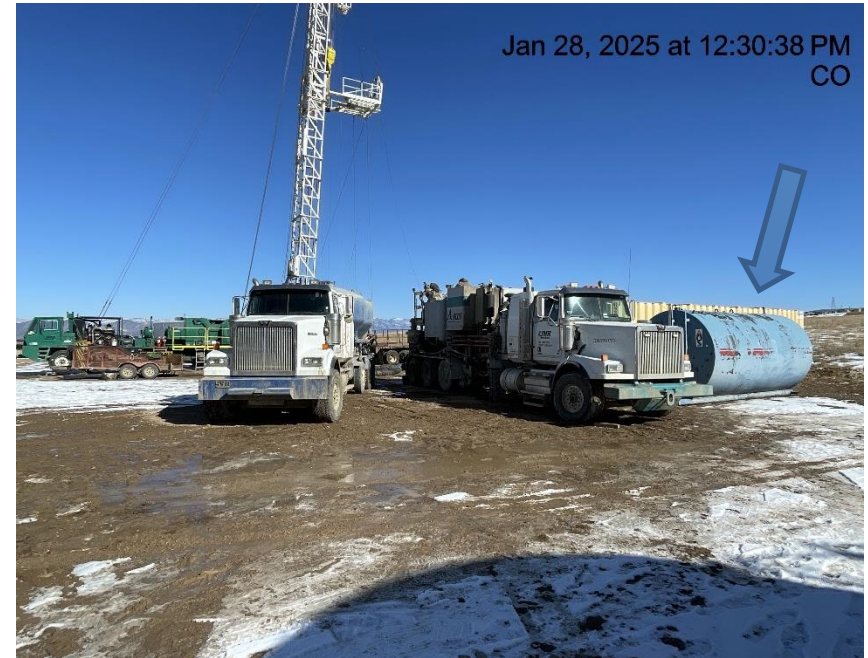
Photo # 1724 Tanks lack secondary containment/failure to comply with COA
