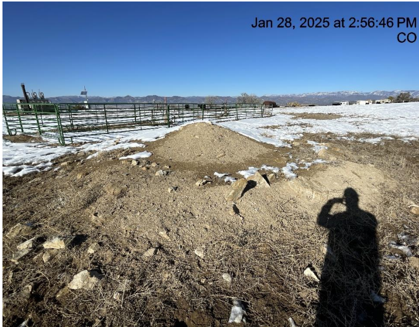
Photo # 2048 Insufficient BMP's around stockpiled soils
