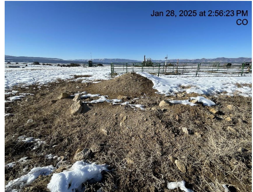
Photo # 2047 Insufficient BMP's around stockpiled soils
