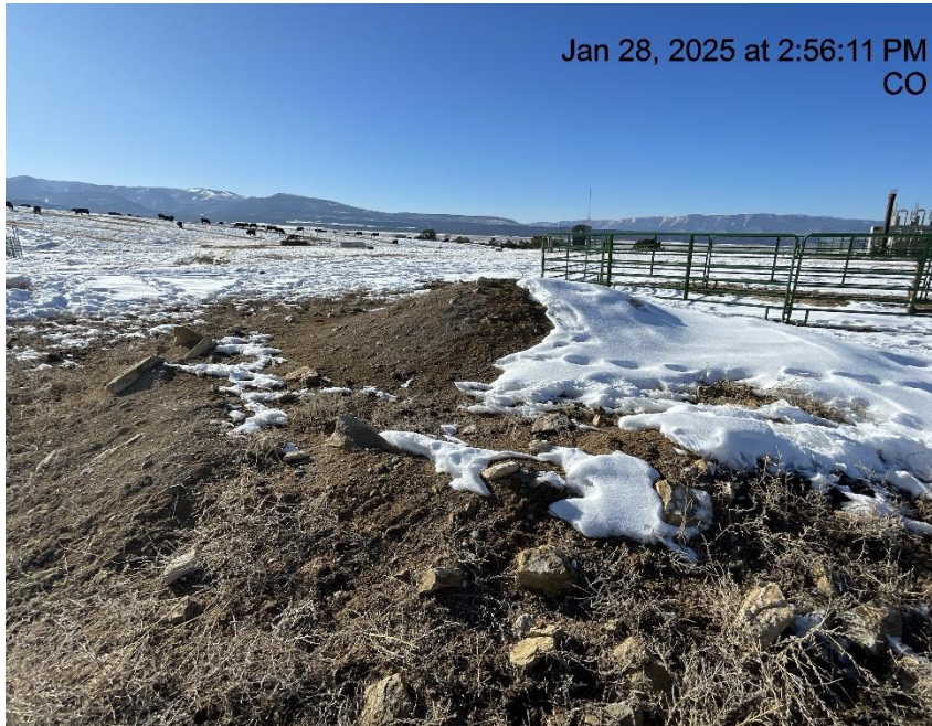
Photo # 2046 Insufficient BMP's around stockpiled soils
