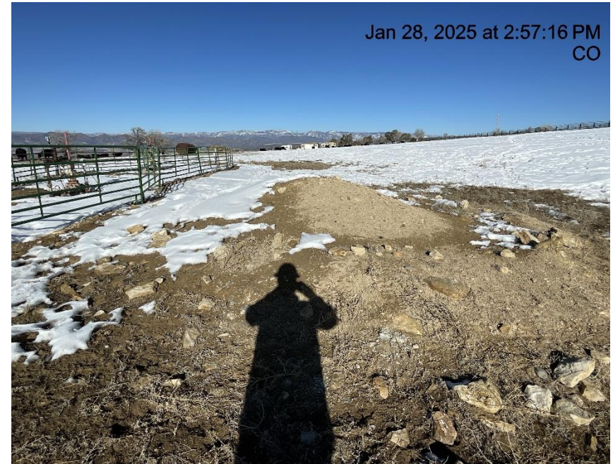
Photo # 2049 Insufficient BMP's around stockpiled soils
