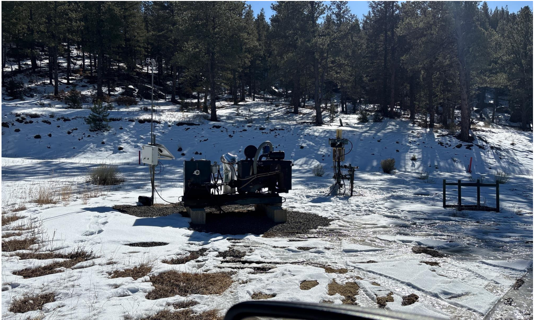
PHOTO 4: TR WELLHEAD AND EQUIPMENT.
