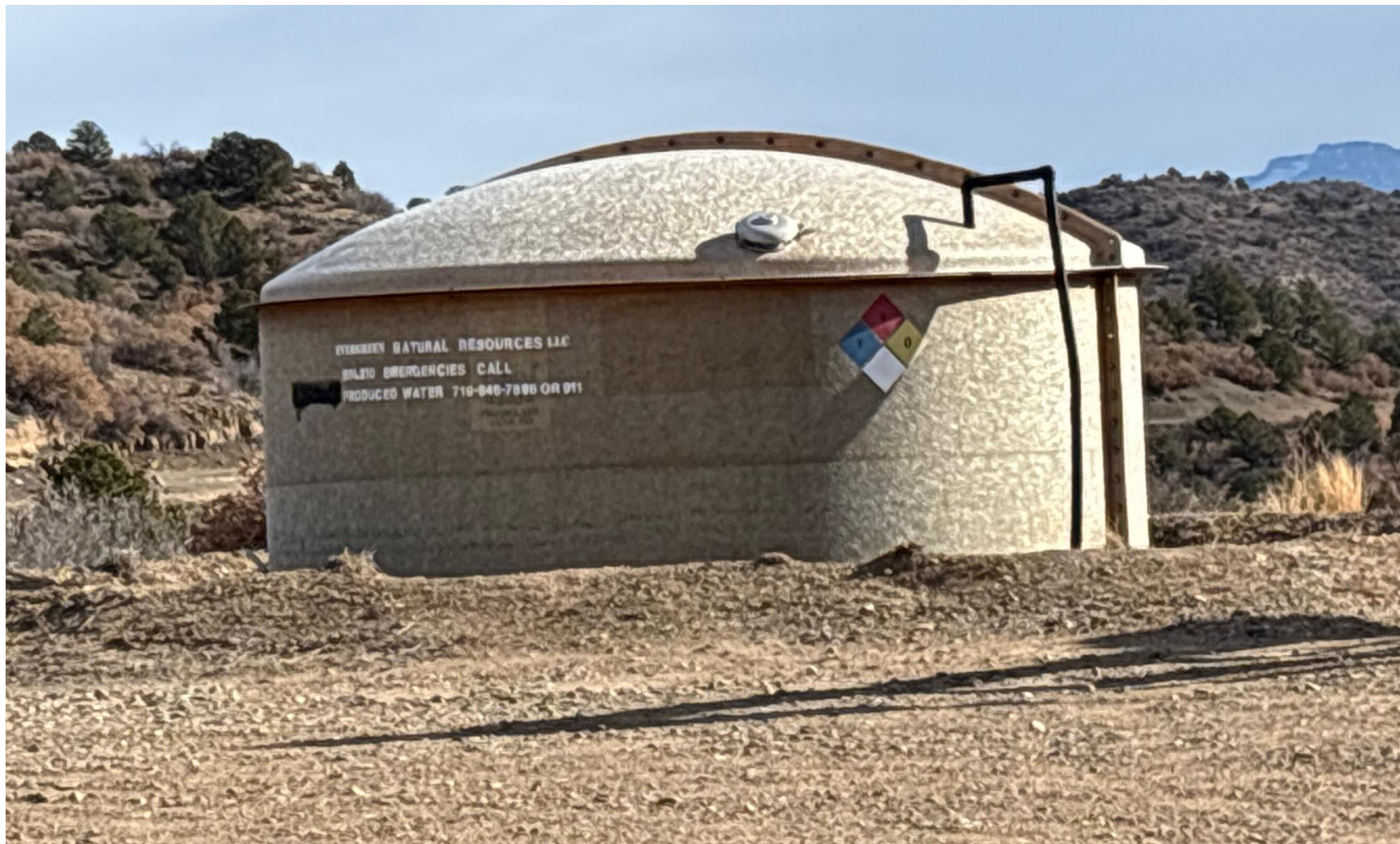
PHOTO 3: PRODUCED WATER TANK BATTERY
