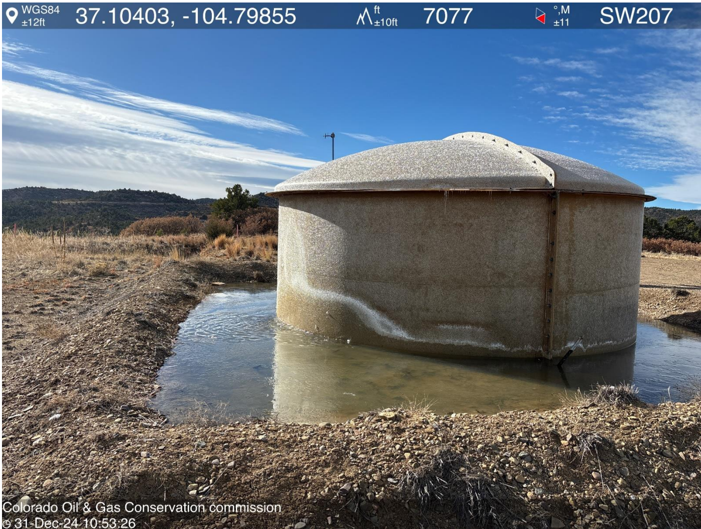
PHOTO 5: PRODUCED WATER TANK IS OVERFLOWING AND SECONDARY CONTAINMENT IS ALMOST FULL (SPOKE WITH ED ROMERO BY TEXT MESSAGE OPERATOR IS SENDING LEASE OPERATOR AND WATER TRUCK). Control and contain spills/releases and clean up per Rule 912.a. CA DATE 1/1/2025.
