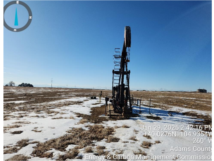
Photo 2 well head and equipment
