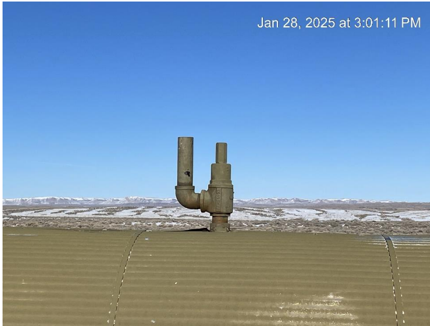
Missing rain cap
