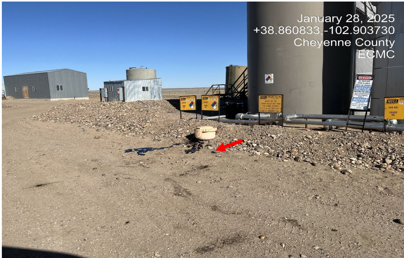
Photo 1. There is oil leaking out of the truck load out at the MUSF #2 TB.
