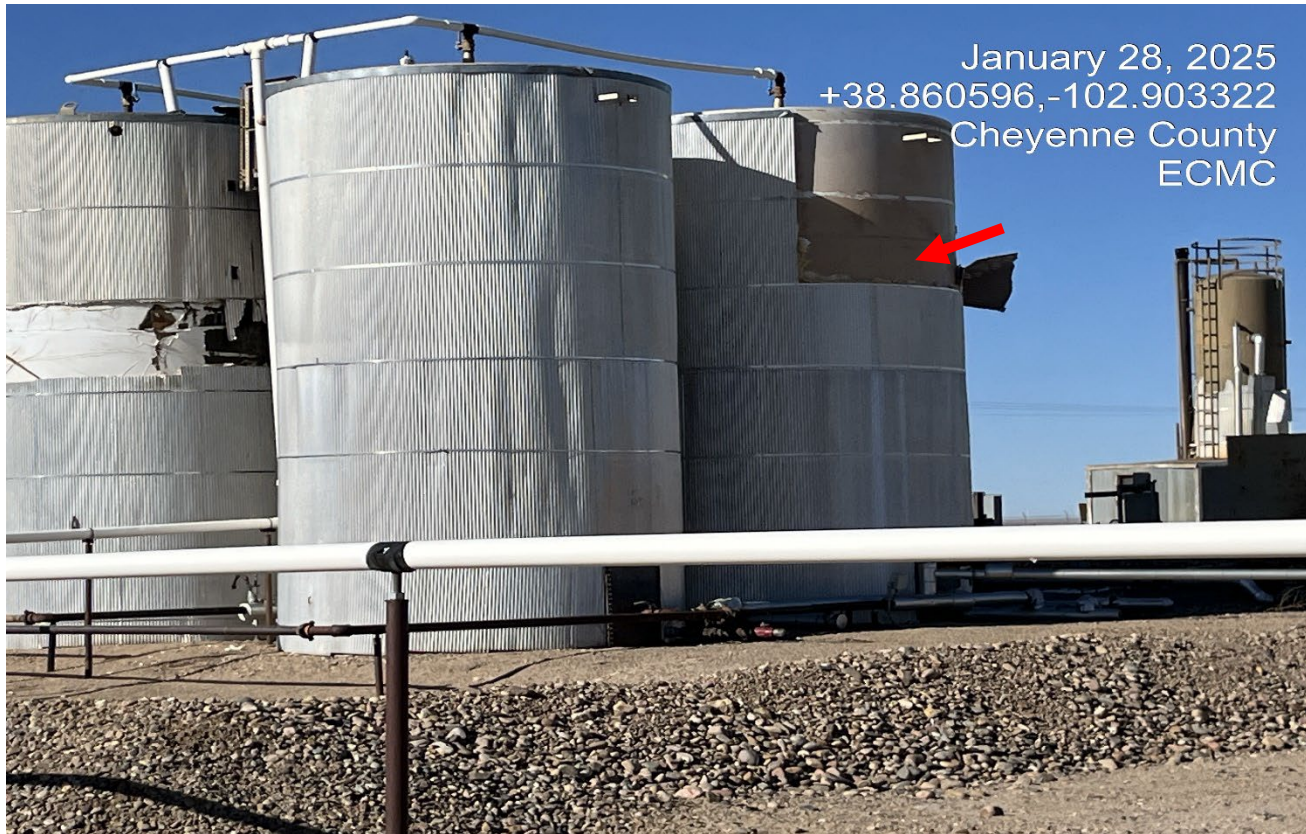
Photo 4. The observed tin and insulation have blown off this tank.
