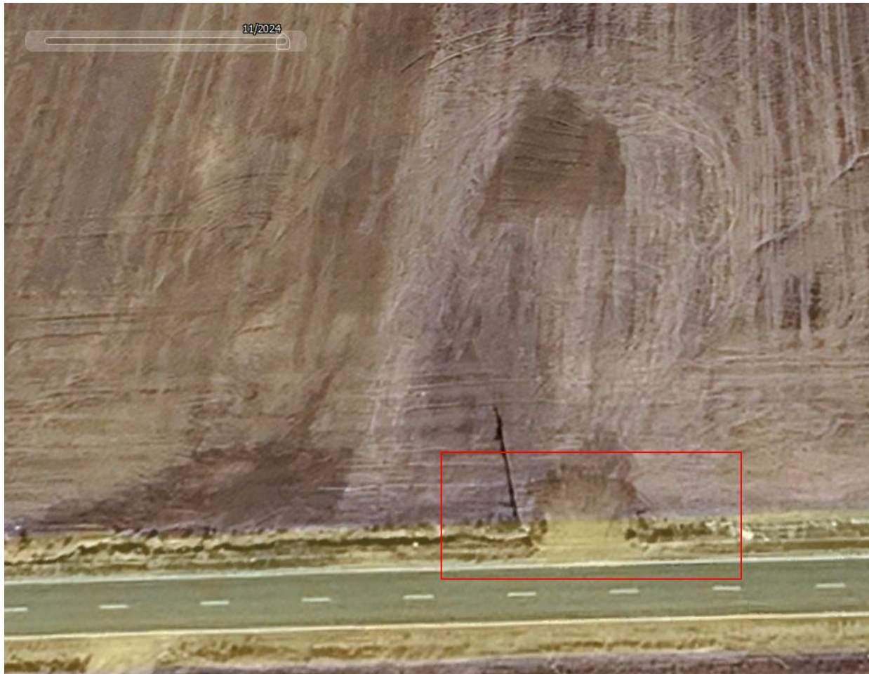
Photo 3. Google Earth aerial imagery (circa 11/2024) illustrating that a portion of the former access point has been reclaimed, but culvert and road base material remain. Additional reclamation activities are required.
