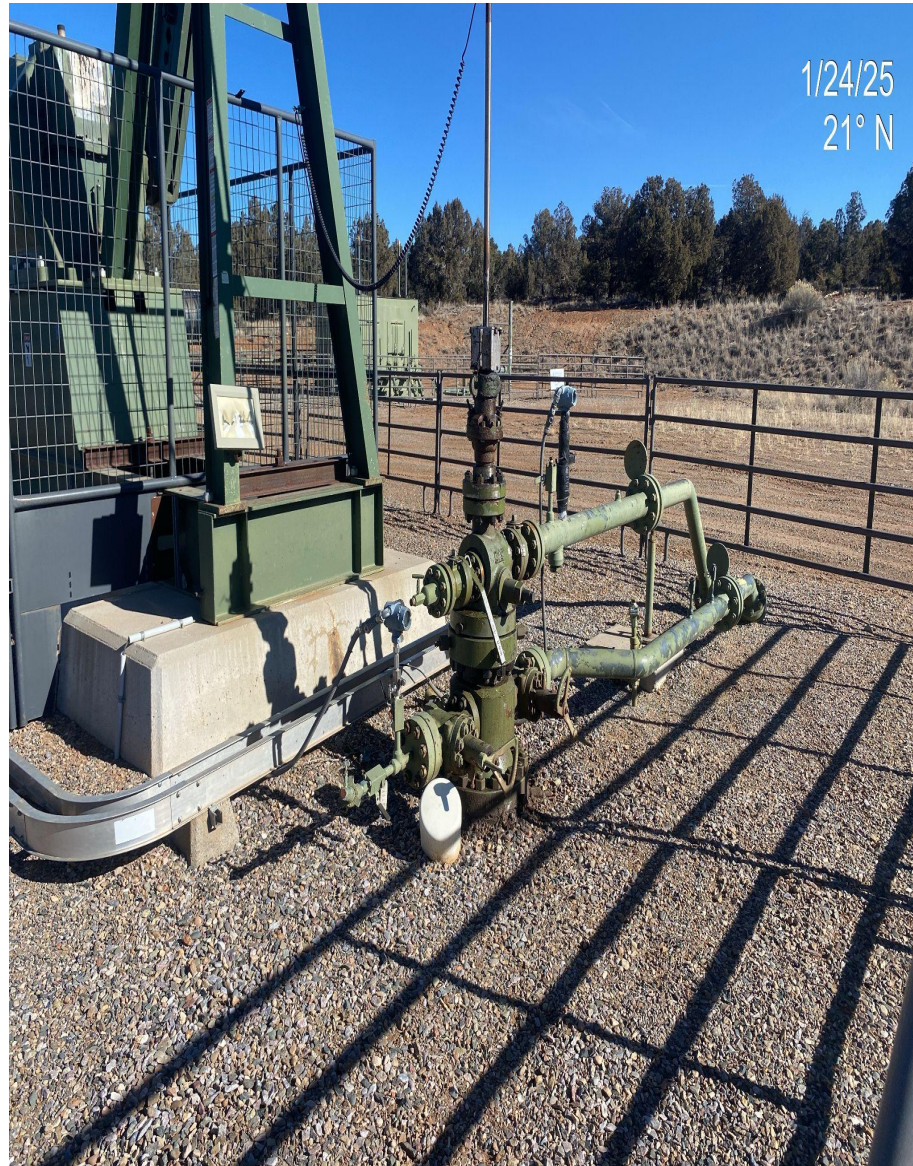
Photo 2. View of wellhead assemblies, no stained soils were observed.
