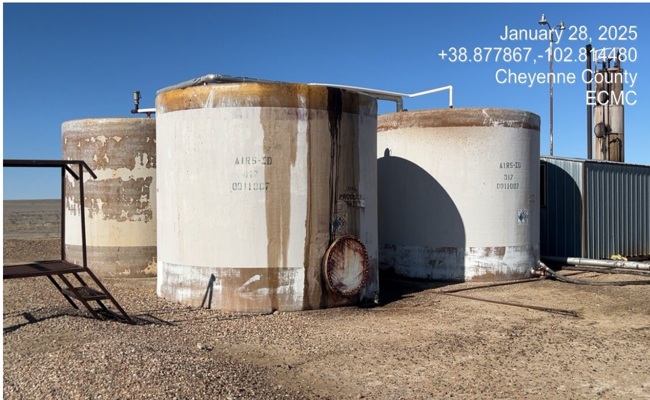
Photo 9. There are signs of a leak at the top of the fiberglass tank.
