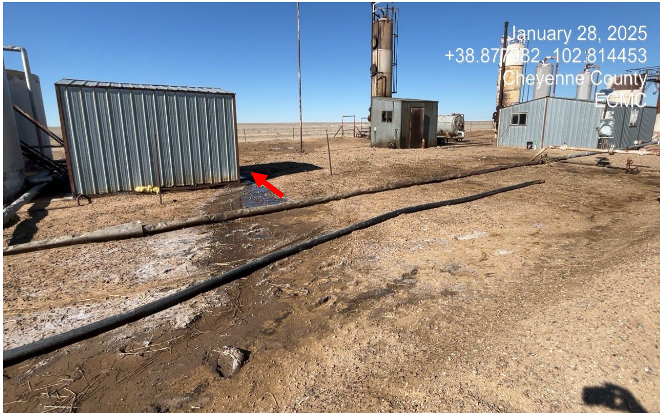
Photo 7. It appears there was also a condensate leak that flowed from the shed at red arrow.
