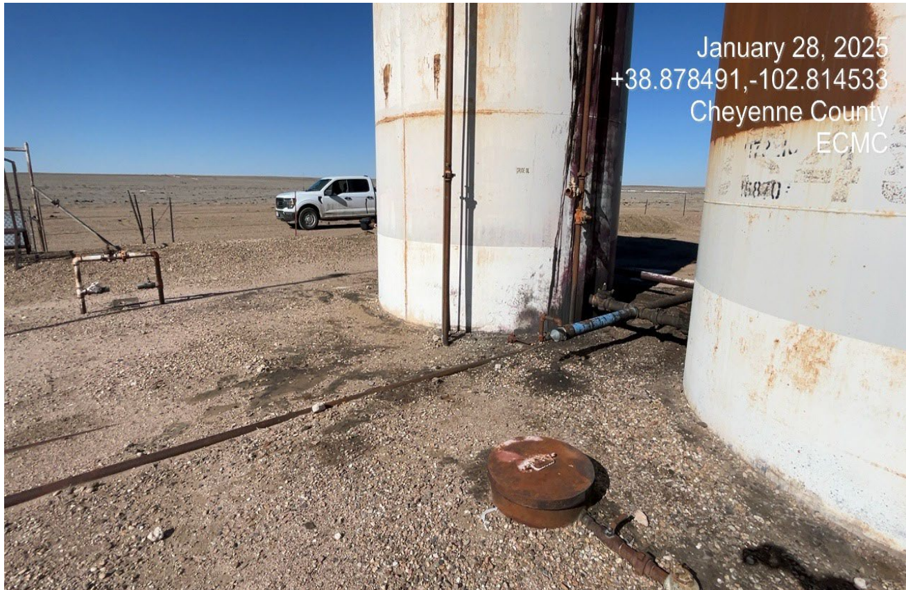
Photo 4. There is oil stained waste between the tanks from a previous spill.
