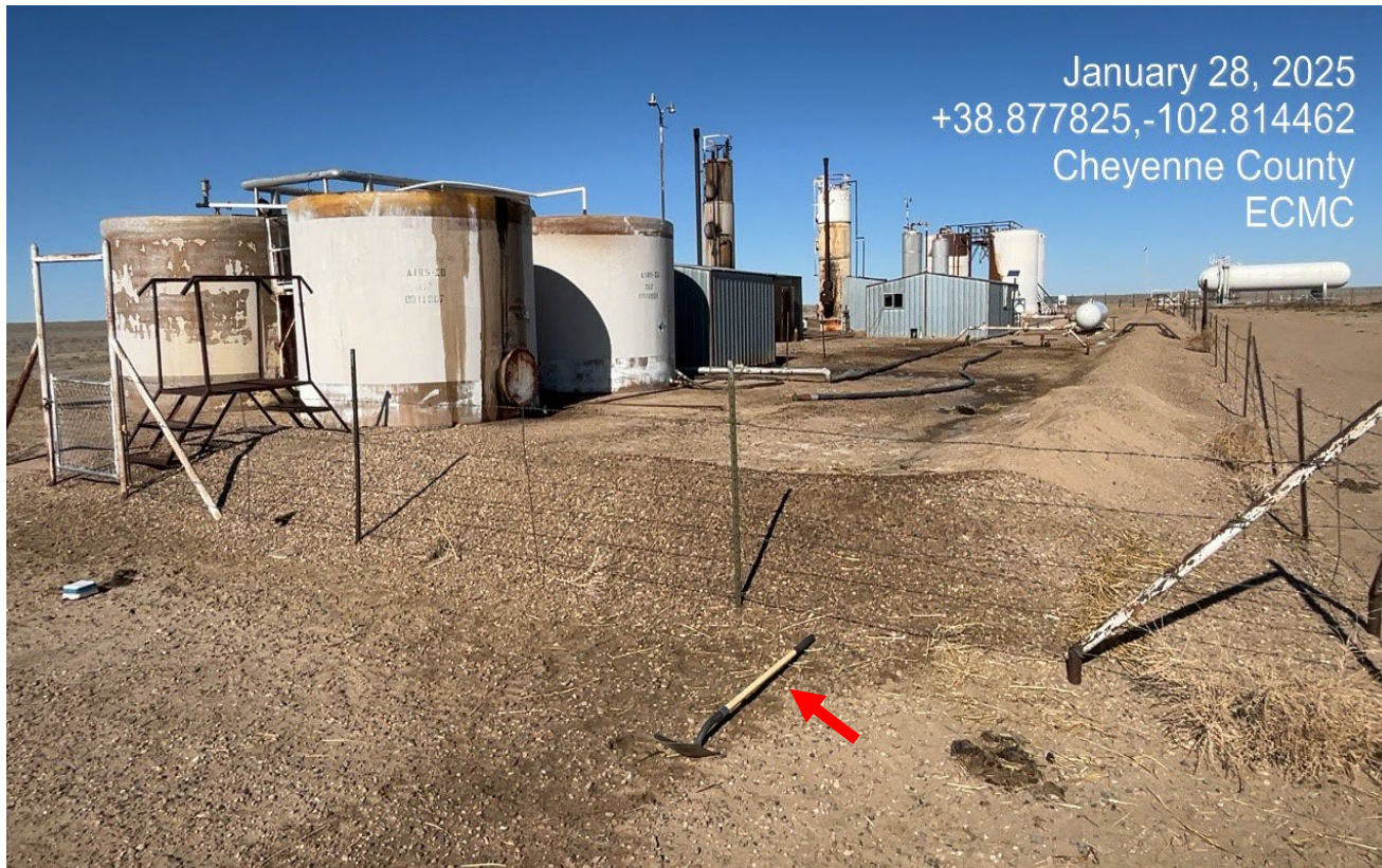
Photo 8. Southeast corner of the location facing northwest toward the tank battery facility. It appears the leak had overtopped this corner with visible impacts shown by the shovel at red arrow.
