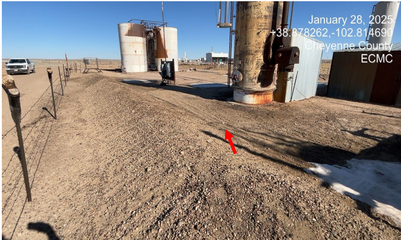
Photo 5. It appears there was a recent spill that occurred near the heater treater. The surface and equipment is blackened from a hydrocarbon mist that recently occurred.
