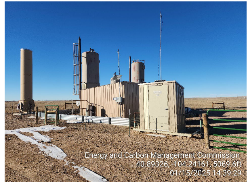
Photo 2 – Heater Treater, Gas Meter and ECD
