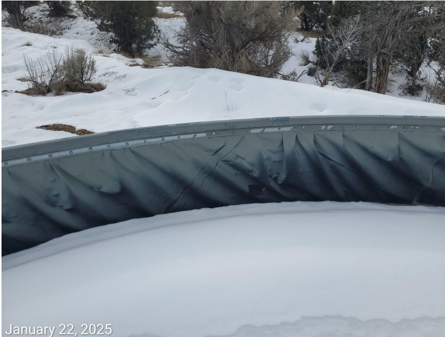
Photo 4: Photo shows holes/tears within the secondary containment liner
