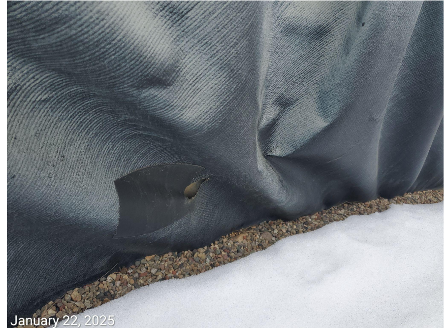
Photo 4: Photo shows holes/tears within the secondary containment liner
