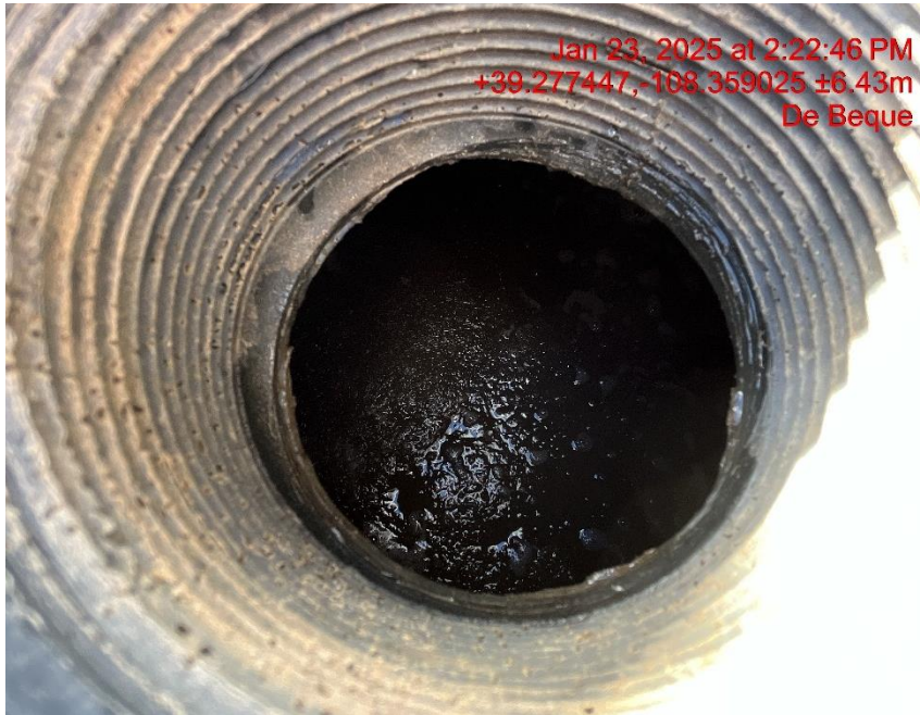
Photo # 3324 Failure to maintain chemical BMP/chemical containment approximately 3/4th full of fluid/not sufficient to contain possible spill
