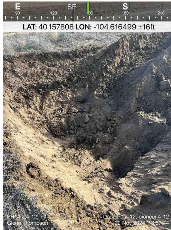
Pothole Sample Location 14
