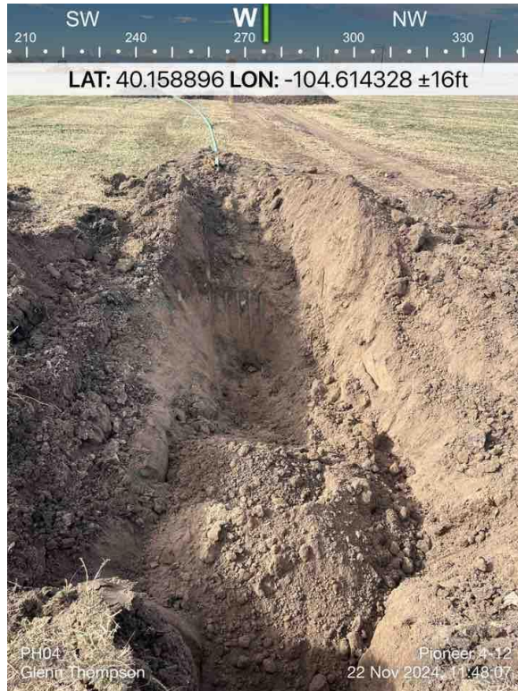
Pothole Sample Location 04
