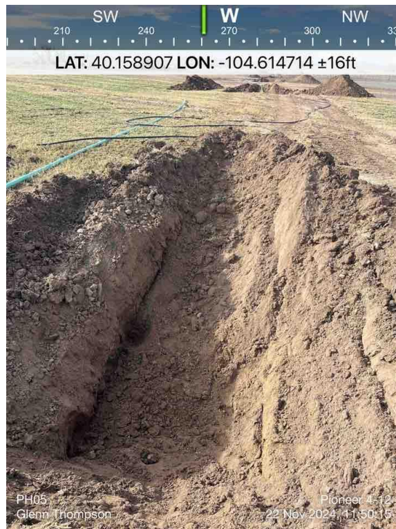
Pothole Sample Location 05
