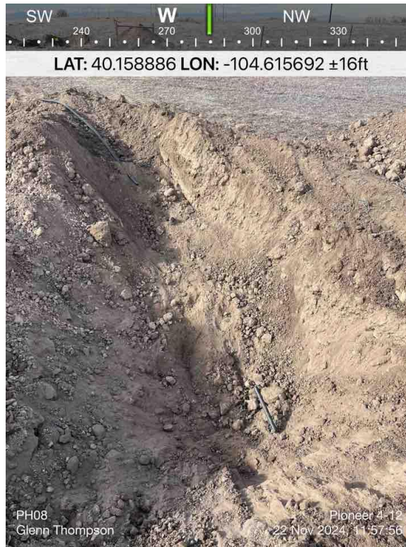
Pothole Sample Location 08
