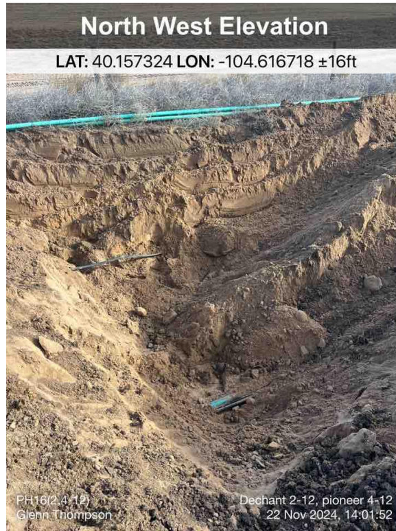
Pothole Sample Location 16
