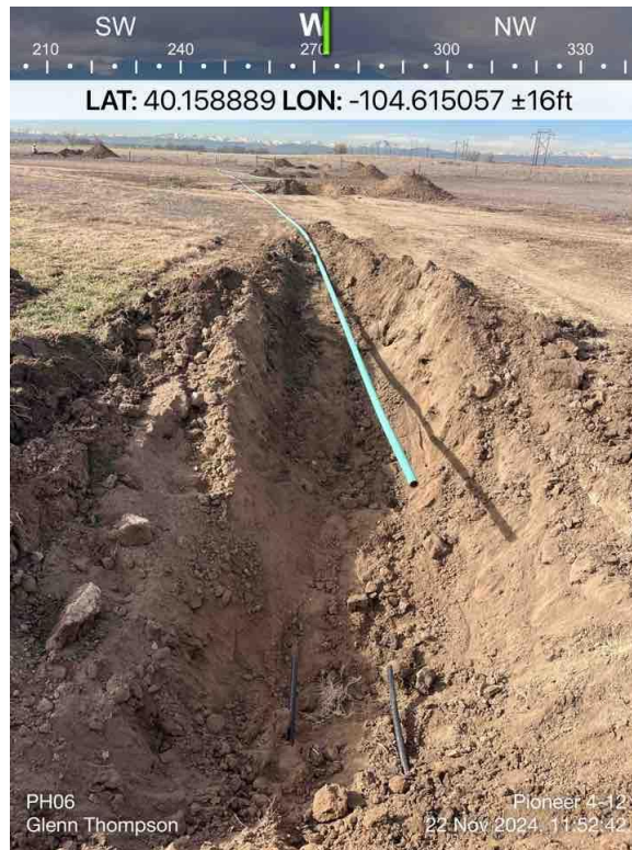
Pothole Sample Location 06
