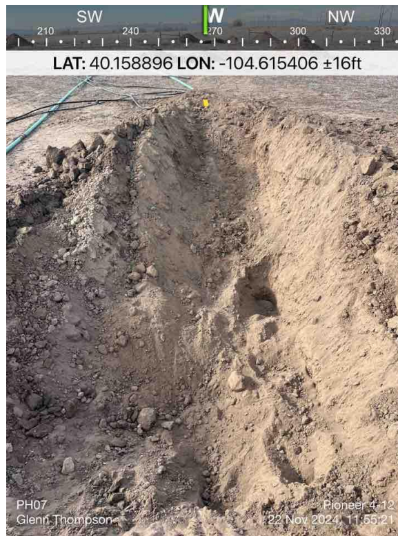
Pothole Sample Location 07
