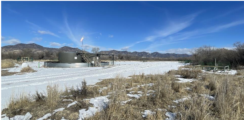
South West corner of location.
