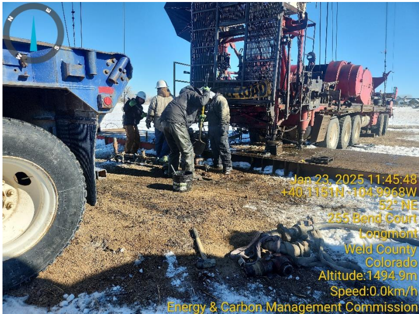
Photo 5 Rig crew prepping WH for cement.
