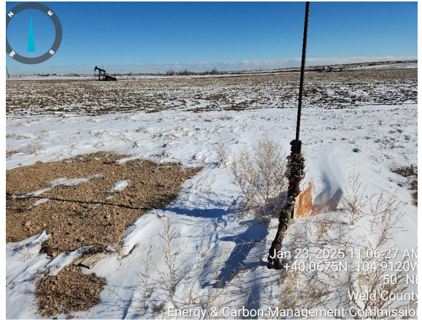
Photo 2 well head and equipment
