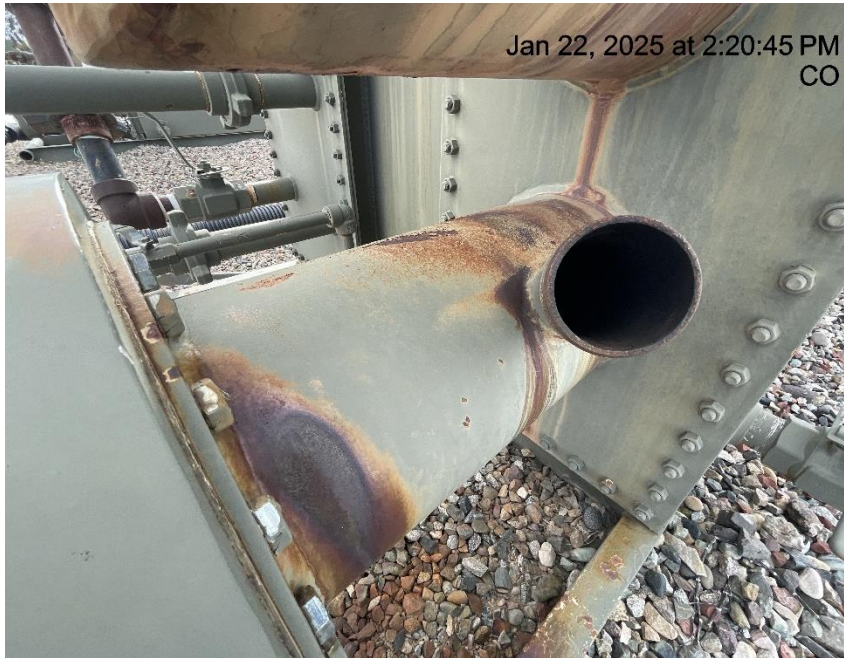
Photo # 807 Burner tube open ended/wildlife hazard /available for entry by wildlife
