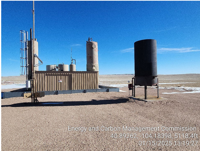
Photo 3 – Heater Treater and ECD
