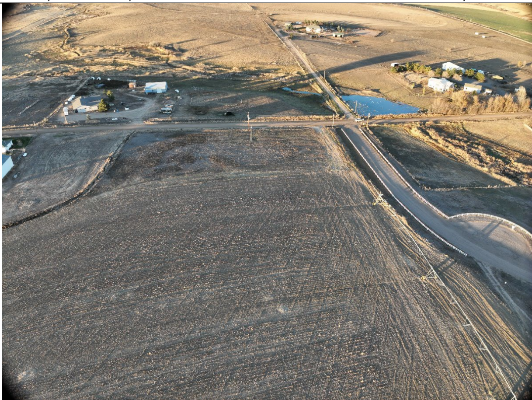
In View – Tank Battery (Loc ID 418911 ), Access Road, Flowline
