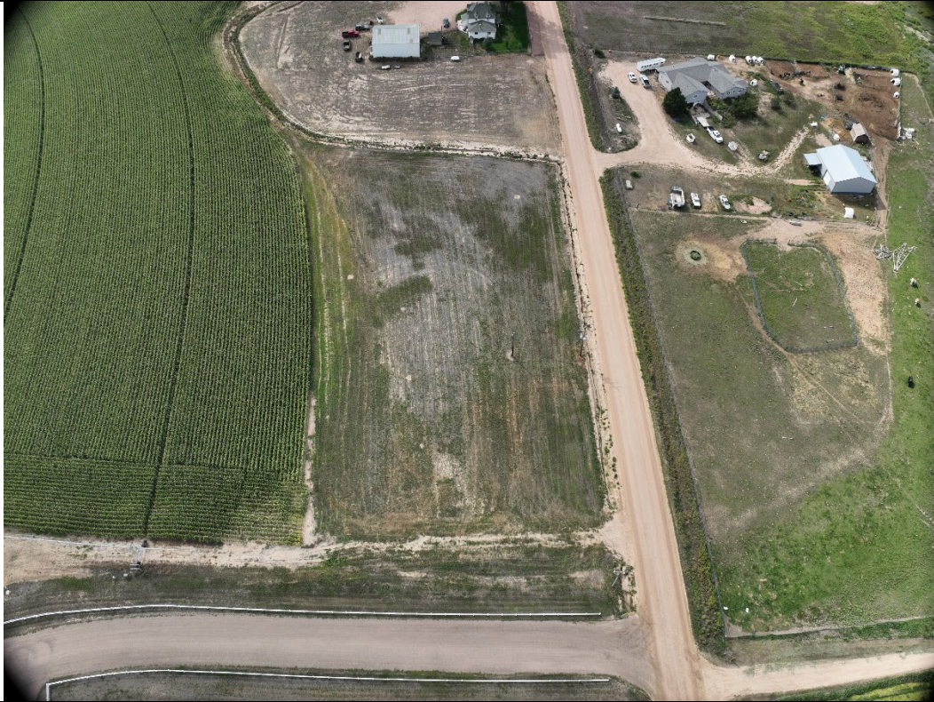
In View – Tank Battery (Loc ID 418911 ), Access Road, Flowline WEST – 40.567285/-104.806659
