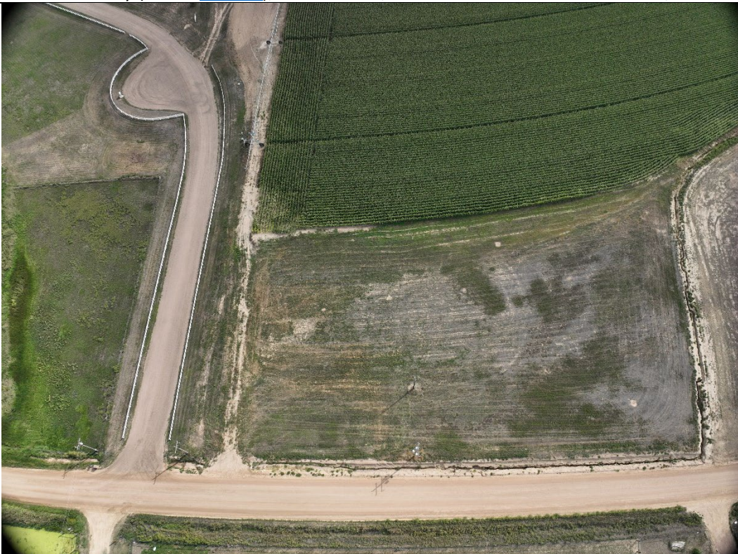
In View – Tank Battery (Loc ID 418911 ), Access Road, Flowline SOUTH – 40.567653/-104.807533
