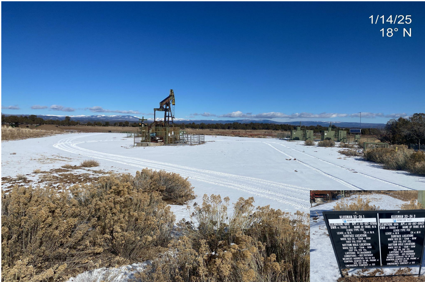
Photo 1. View of well pad from the access point facing center.
