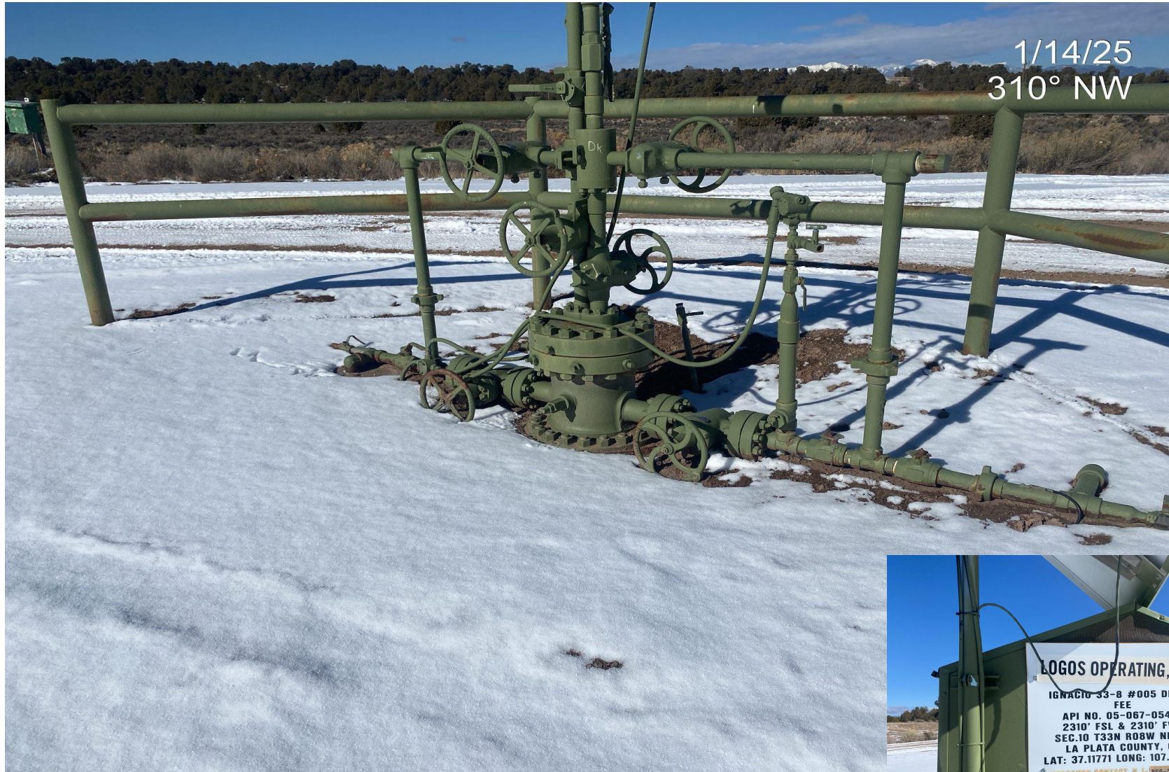
Photo 1. View of wellhead assembly.
