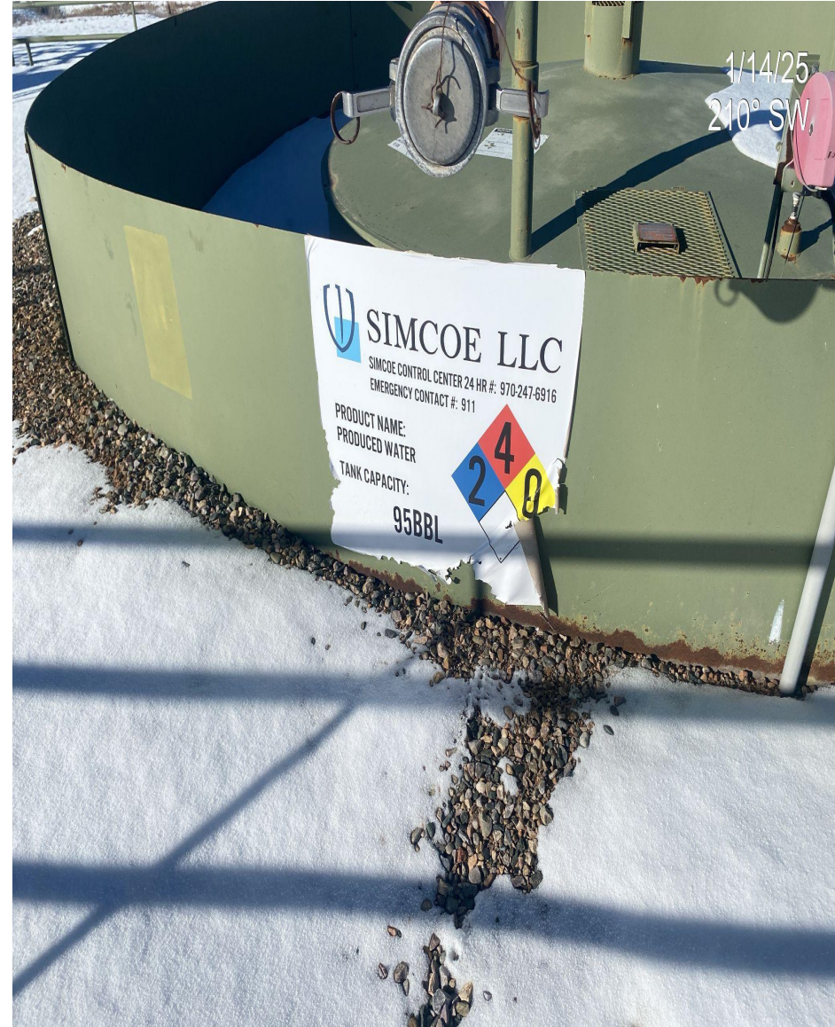
Photo 3. Signs/Labels at separator and produced water tank are deteriorating, future maintenance is advised.
