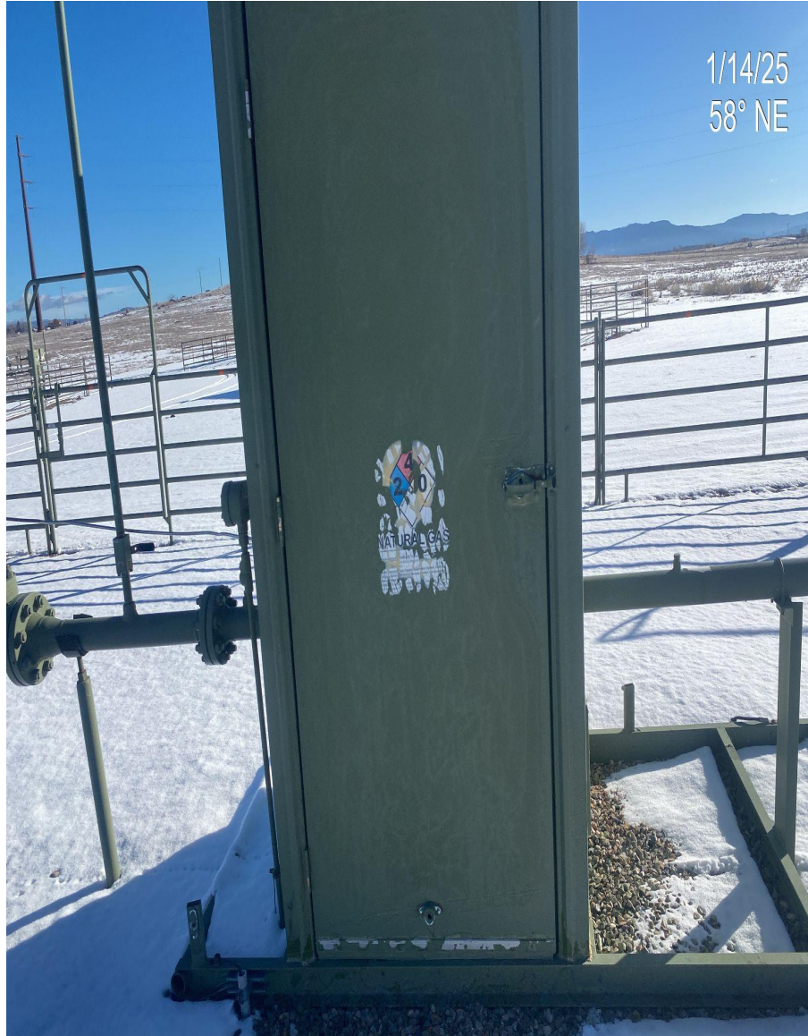
Photo 3. Signs/Labels at separator and produced water tank are deteriorating, future maintenance is advised.
