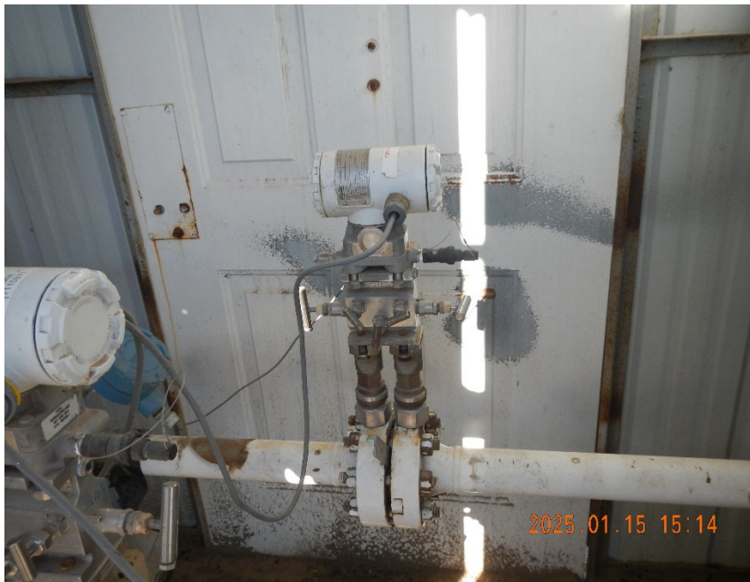
7. Gas meter inside meter shed.
