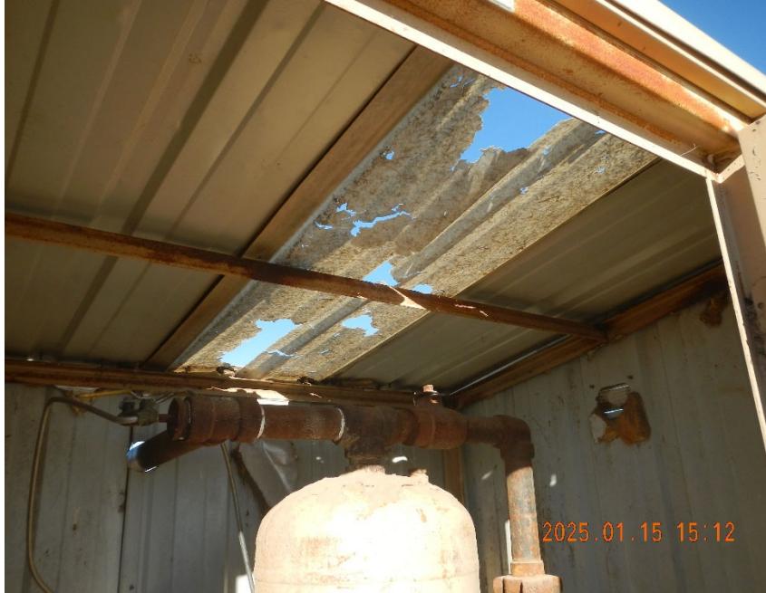
5. View of roof damage to separator shed.
