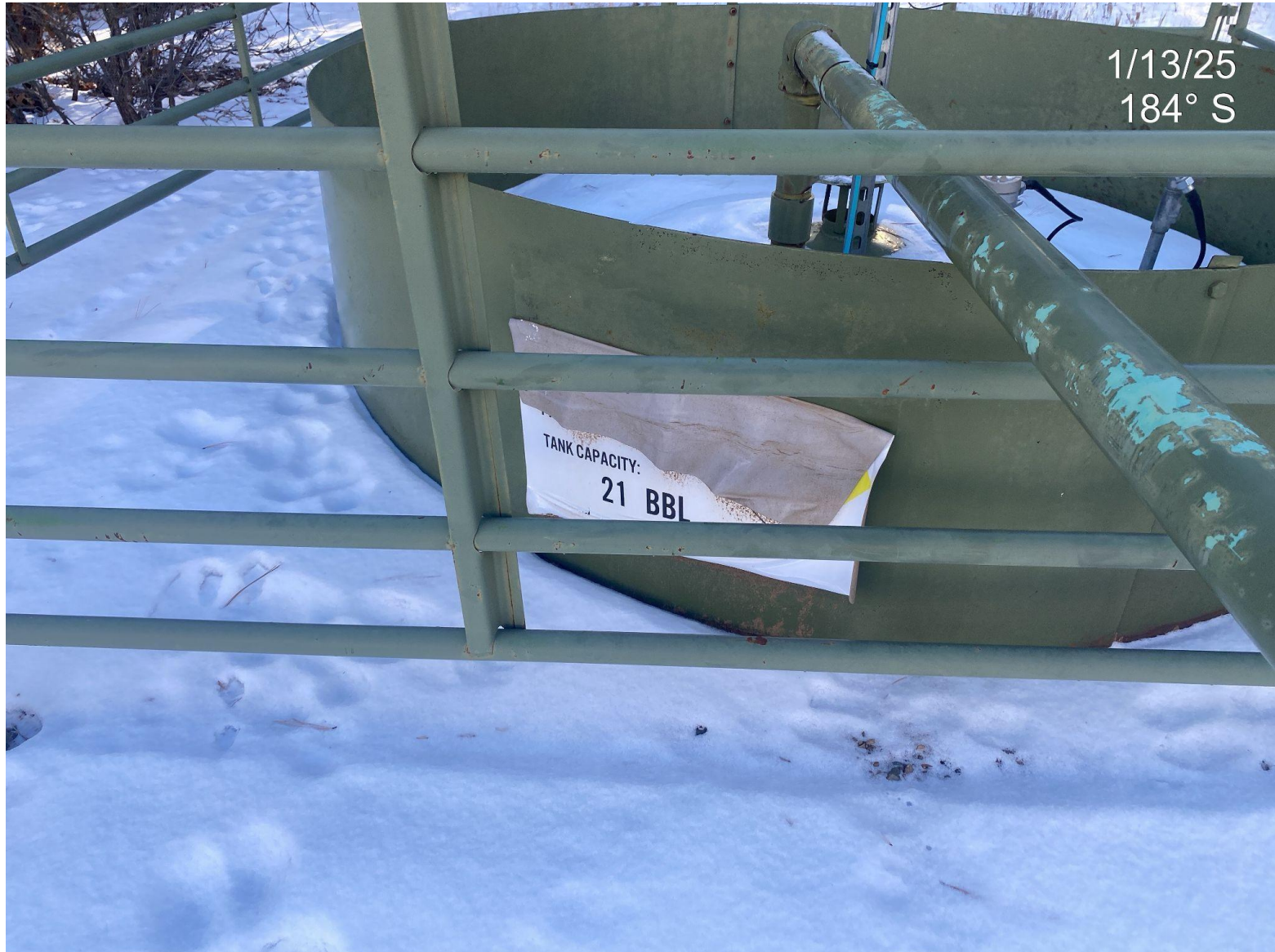
Photo 2. Produced water tank label is peeling and no longer legible.
