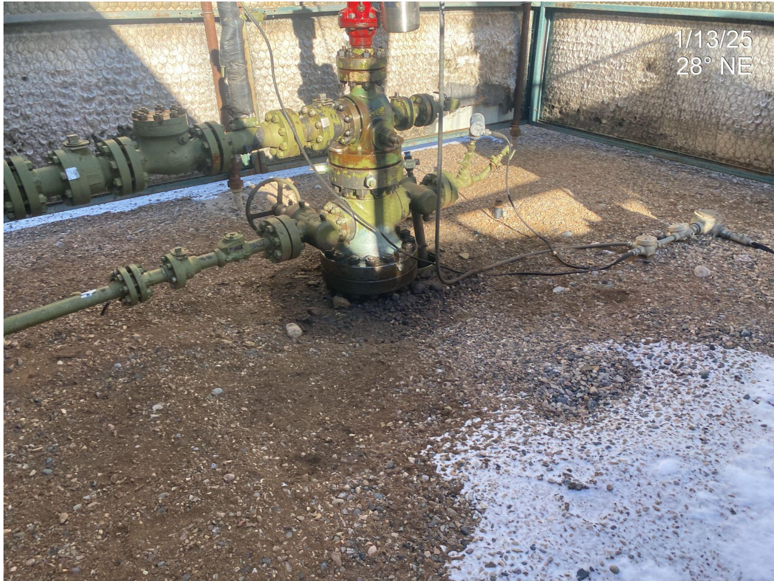
Photo 3. Impacted surface material observed at well head.
